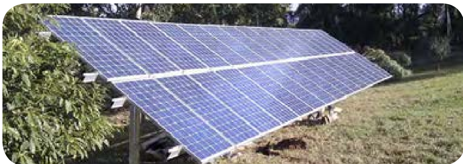
6kW Groundmount Solar Array
