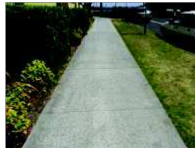
"Very Good" condition footpath
