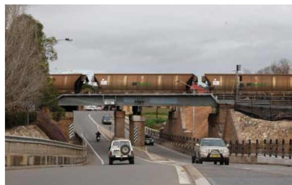
Muswellbrook Shire has well maintained road and rail infrastructure.
