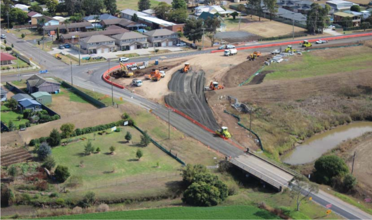
This new intersection at Crinoline Street in Denman improves safety
