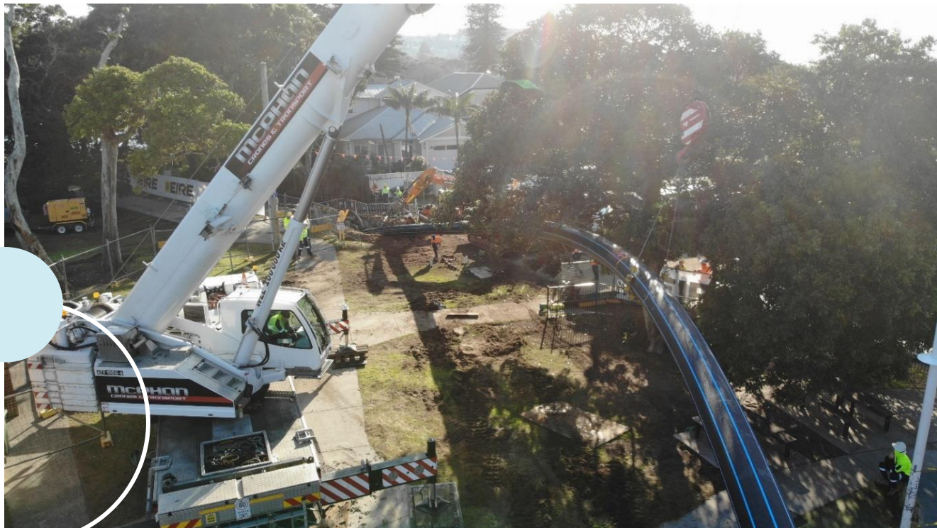
Avoca side with pipe string
