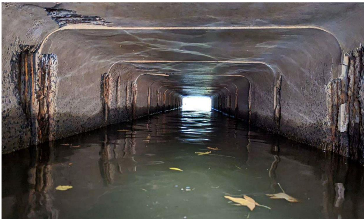
Figure 13: 317 Lakedge Avenue culvert looking downstream prior to replacement
