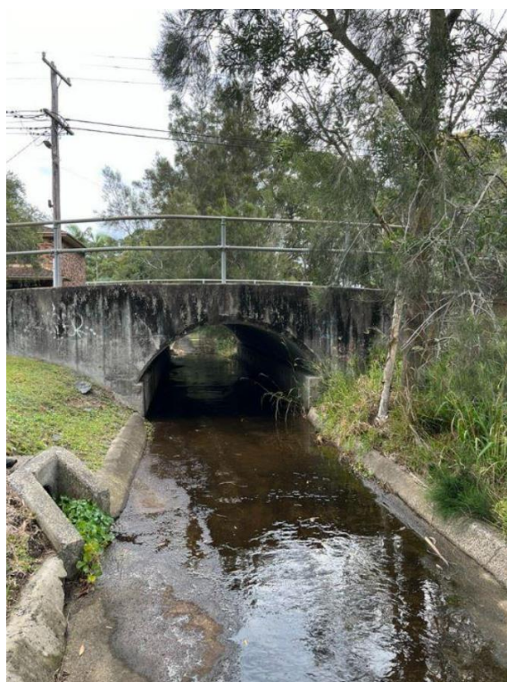
Figure 15: Rushby Street culverts looking upstream and showing the structural failure in the arch
