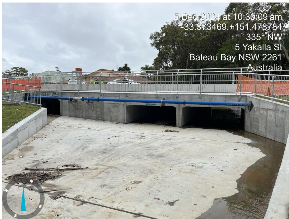
Figure 12: Yakalla Avenue culvert looking upstream following project completion
