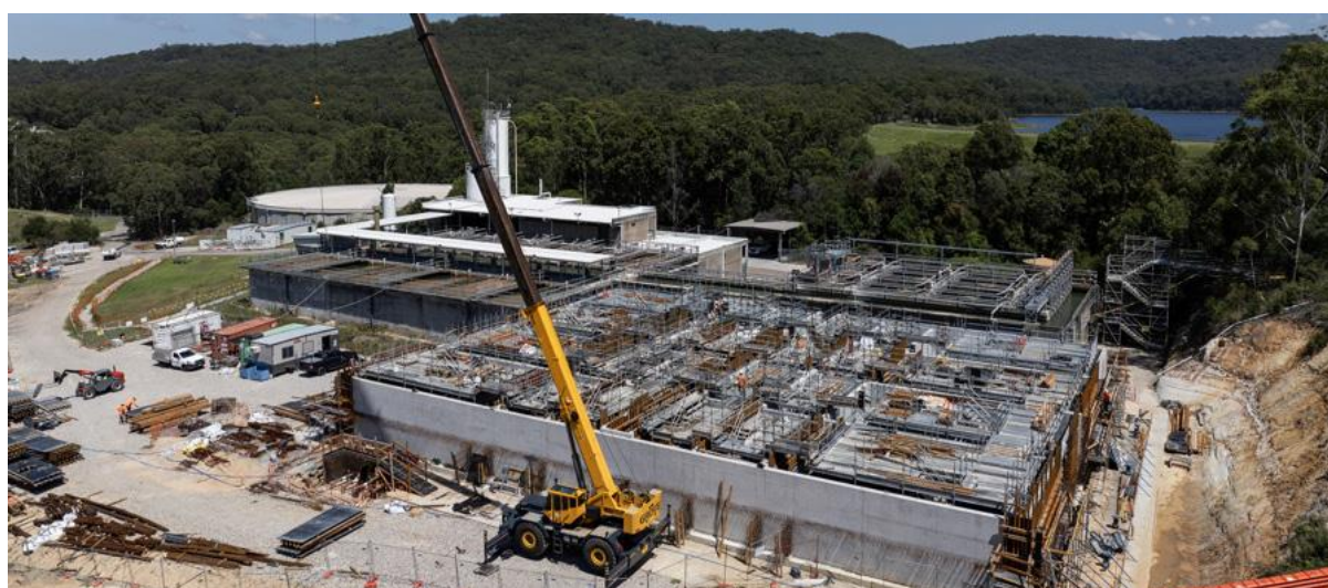
Ongoing construction of the new dissolved air floatation tanks.
