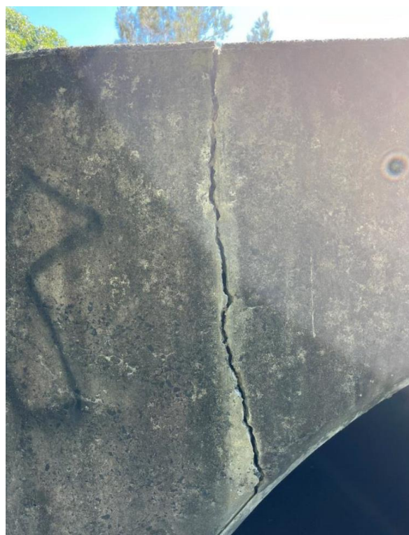
Figure 15: Rushby Street culverts looking upstream and showing the structural failure in the arch
