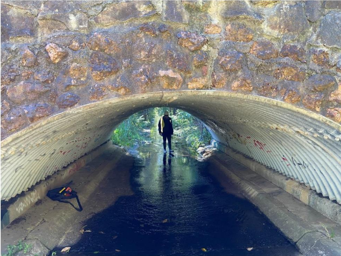
Figure 11: Yakalla Avenue culvert looking downstream prior to replacement
