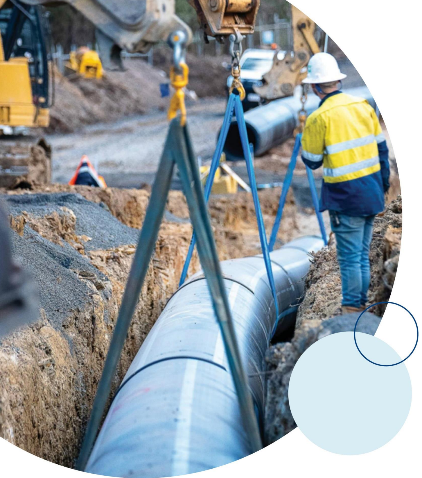
Figure 4: Council laying pipework
