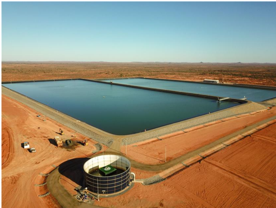
Figure 8: WaterNSW's bulk water storage facility
