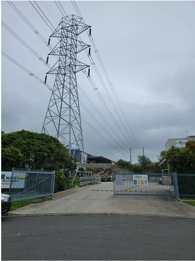
Photo Description: Easement at Denoci CI
