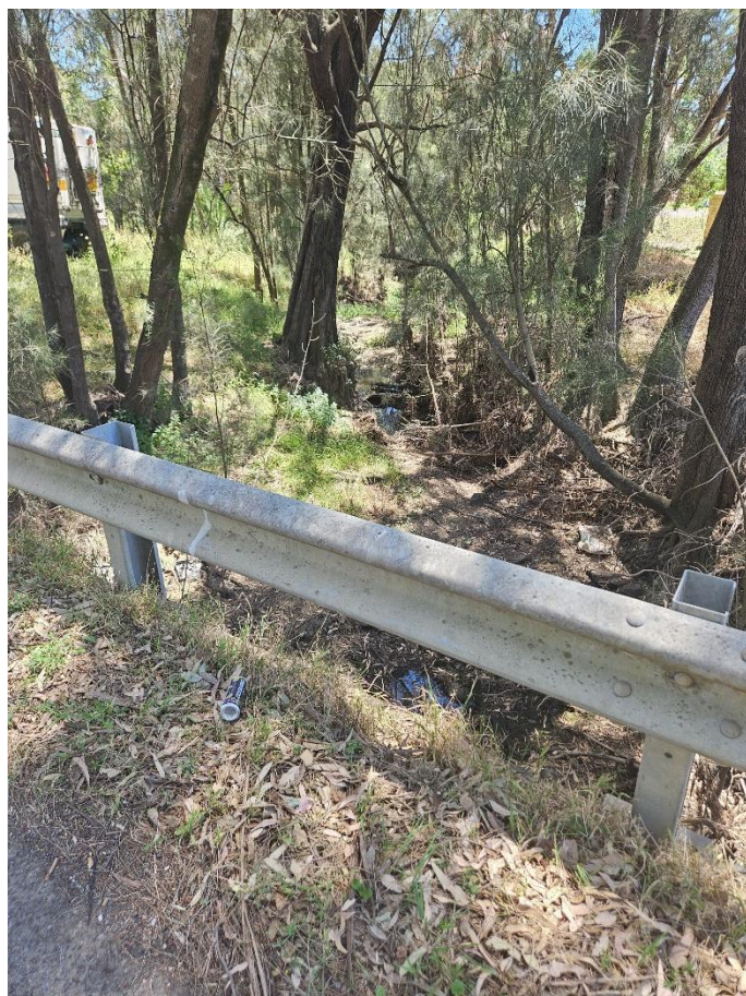
Photo Description: Electricity power lines x2 and steel busines
