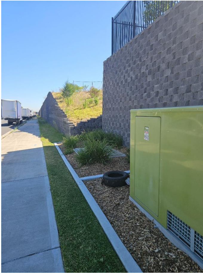
Photo Description: Approx. 8m high retaining wall, facing north along Johnston Cr
