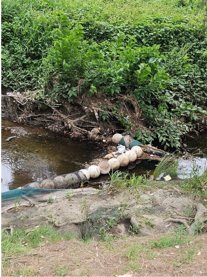
Photo Description: Sediment / litter control
