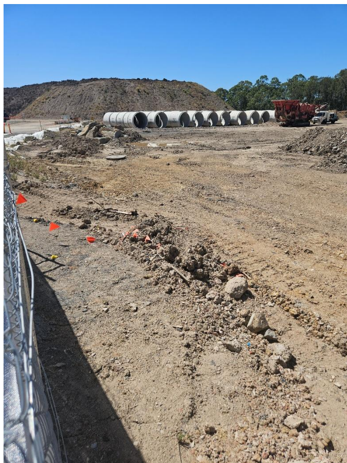
Photo Description: Oakdale East construction site retaining wall and cutting
