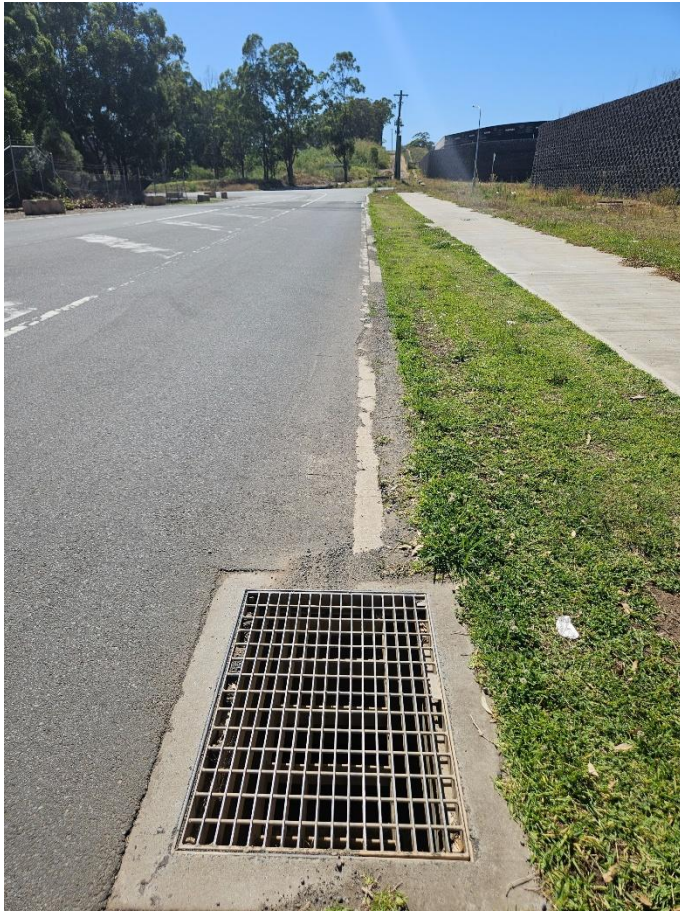
Photo Description: The sewerage main, facing east
