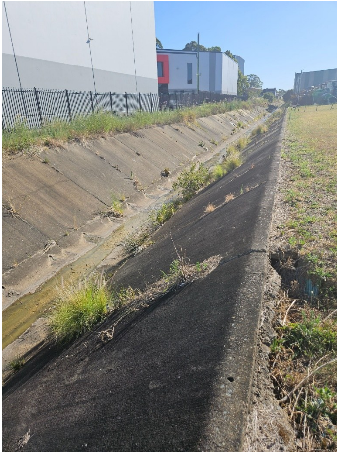
Photo Description: Concreted drainage channel flowing north to the Victoria St two lane roundabout
