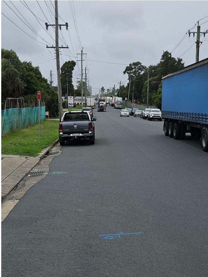
Photo Description: Gently undulating topography
