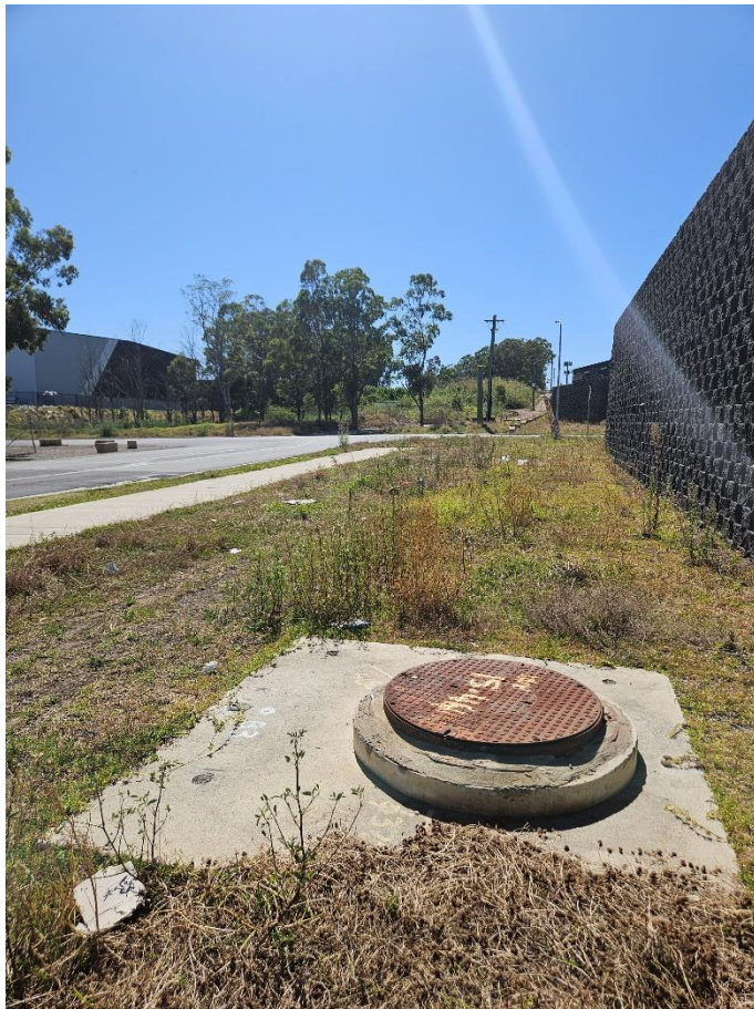
Photo Description: The sewerage main, facing west
