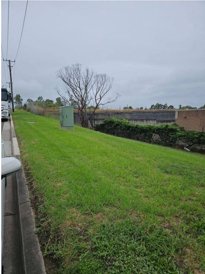
Photo Description: 10m retaining wall
