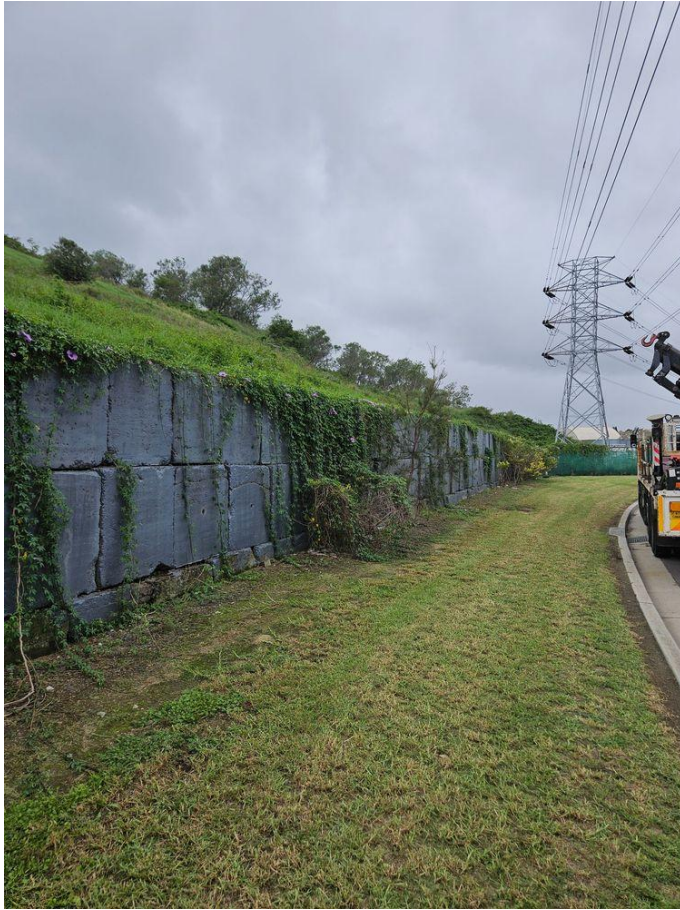
Photo Description: Vegetated stockpile with retaining wall (2m).
