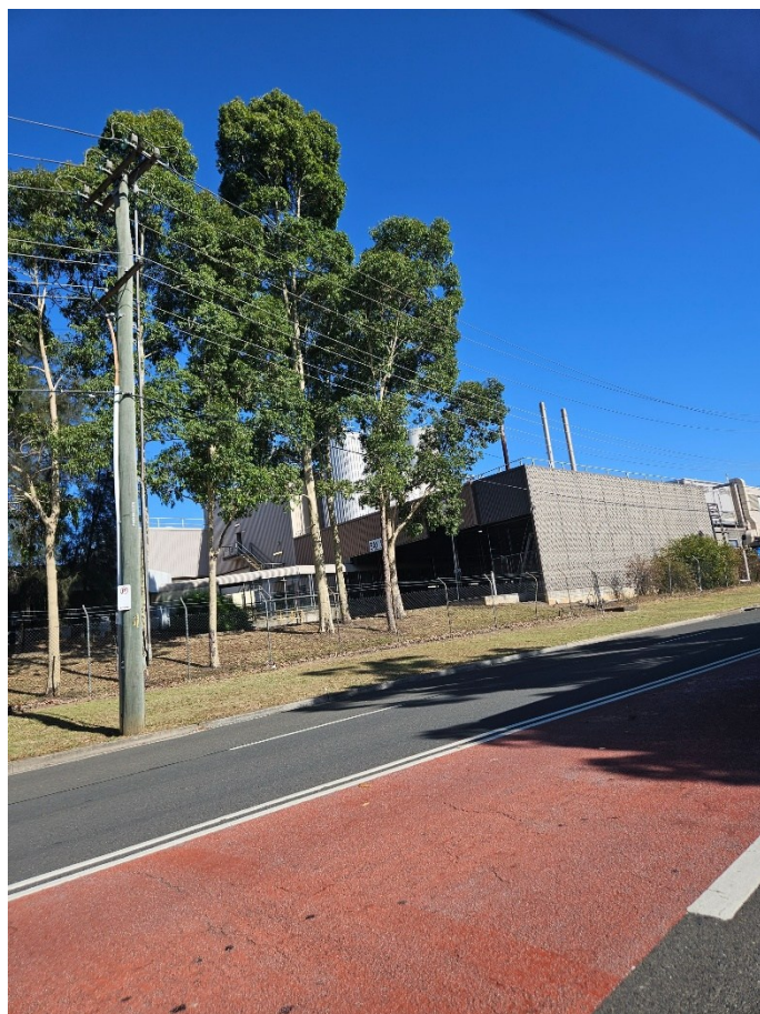
Photo Description: Chemical / gas storage at ABC Tissue Products
