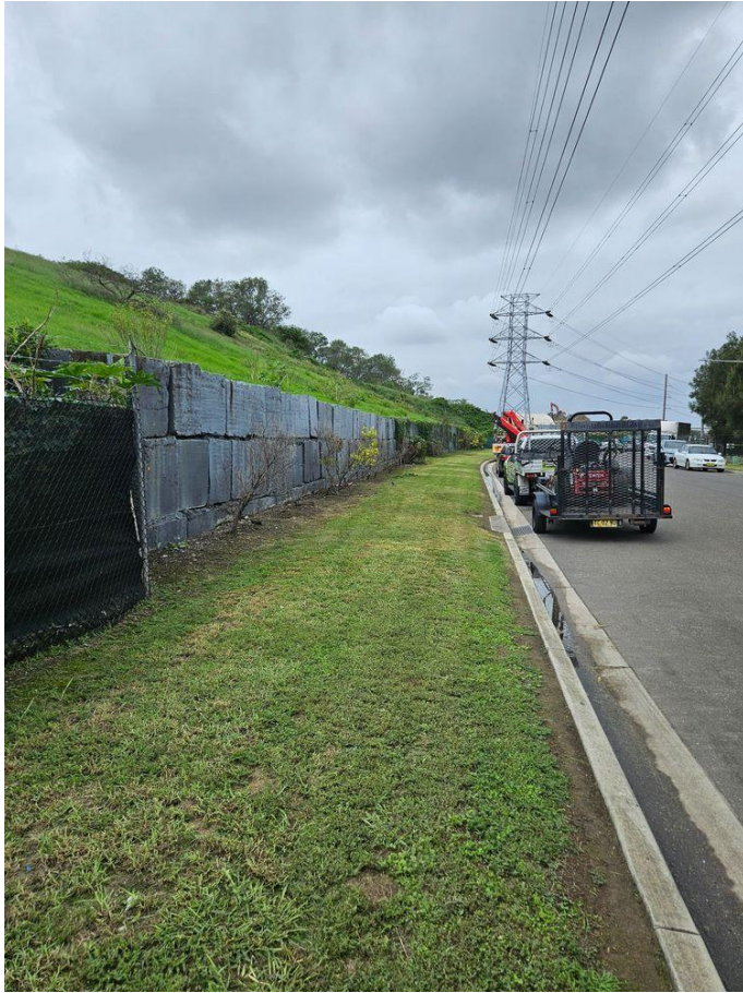
Photo Description: Filling at ECORR.
