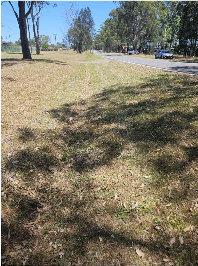
Photo Description: Reedy Ck looking north to Burley St with 4 circular culverts
