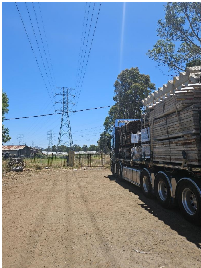
Photo Description: Electricity power lines x2
