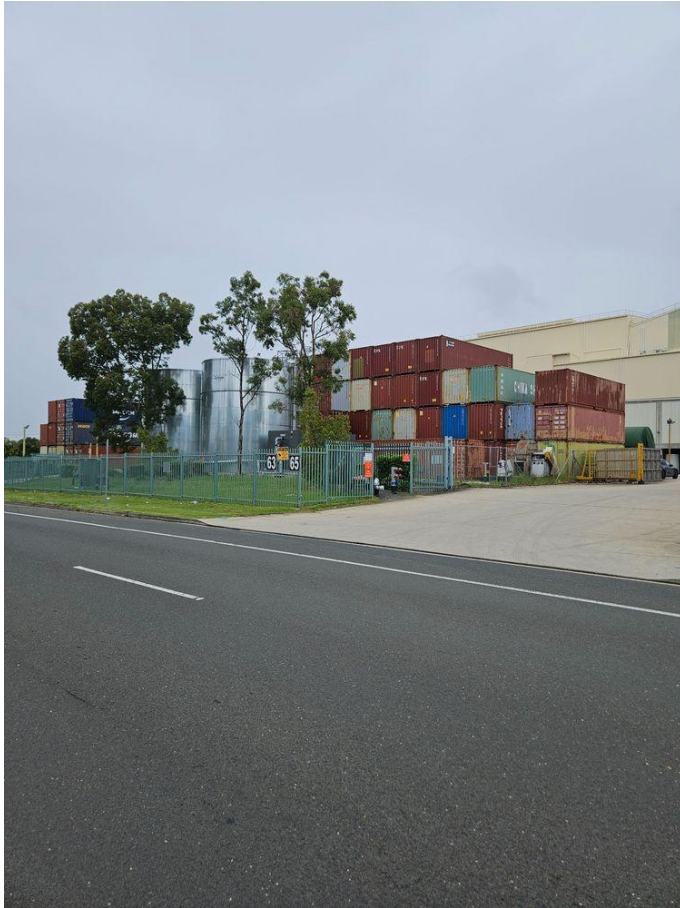
Photo Description: ASTs and shipping container storage
