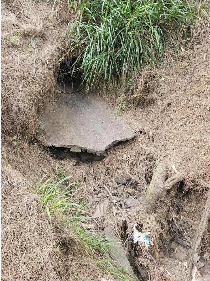
Photo Description: Stormwater outlet
