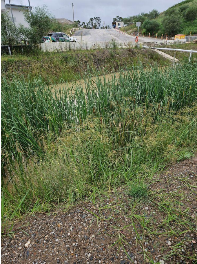
Photo Description: Onsite water body and cut & fill works at ECORR.
