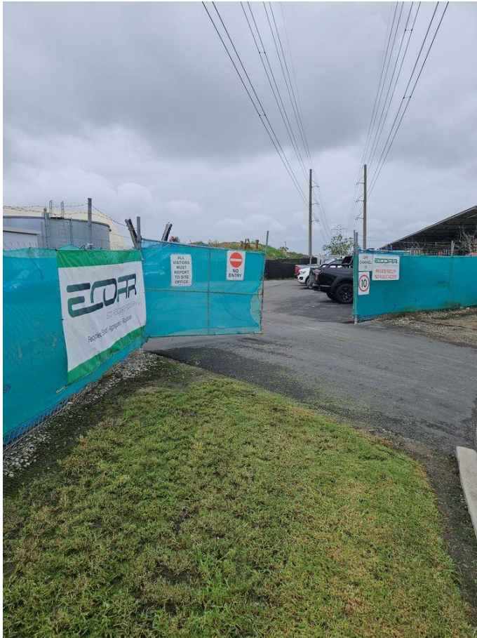
Photo Description: Easement at McKay Rd facing east. ECO RR - ECO RESOURCE RECOVERY, recycled sand, aggregates and road-bases. Multiple large stockpiles (>5m height), storage of large truck tires.
