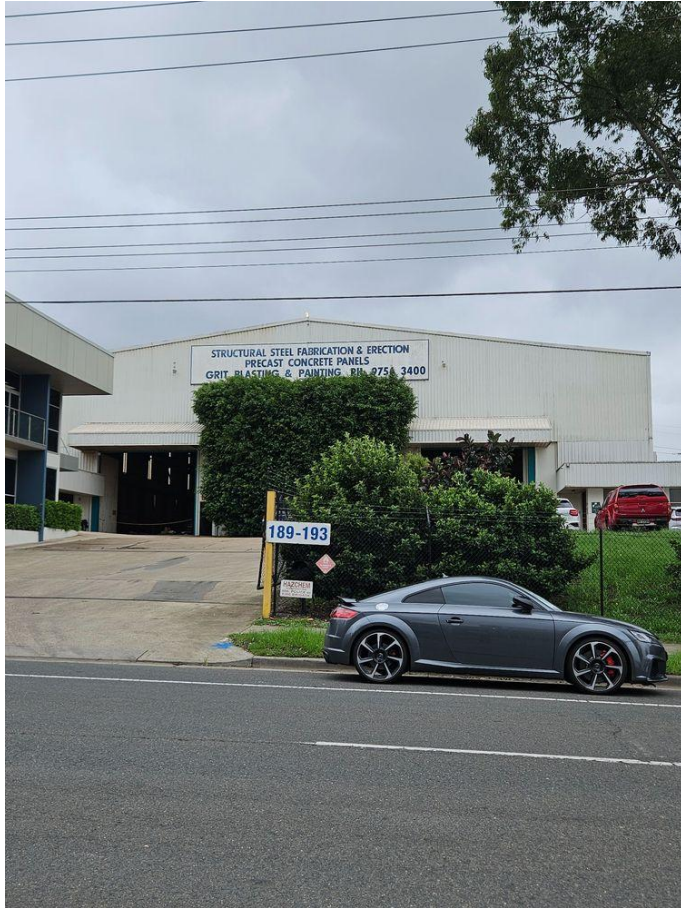
Photo Description: Steel fabrication at a commercial property
