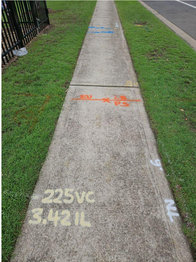
Photo Description: Underground services
