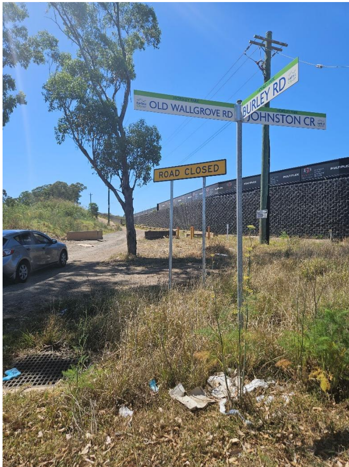
Photo Description: Oakdale aeast construction including stockpiling and pipeline.
