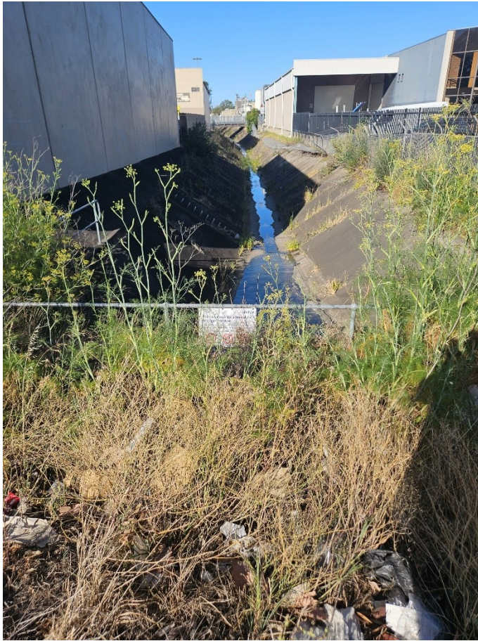
Photo Description: Stormwater drainage channel, Southwest facing
