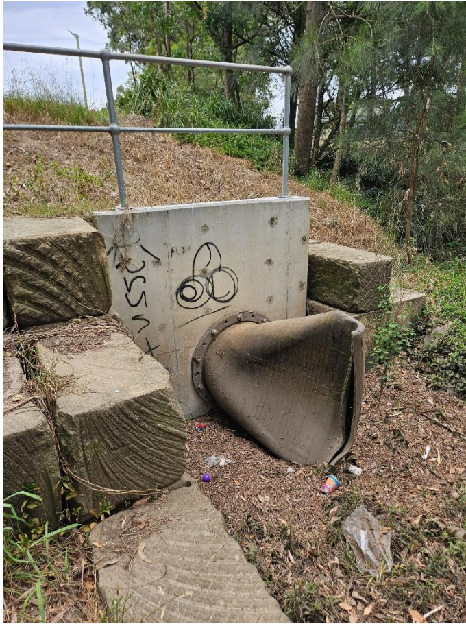
Photo Description: Historical stormwater outlet
