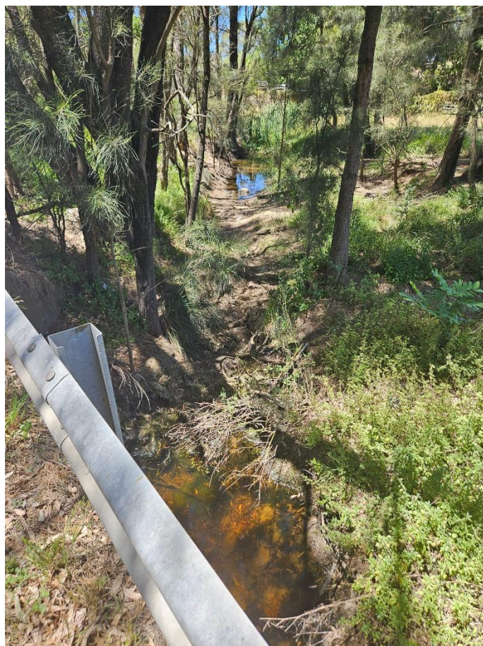
Photo Description: Reedy Ck and Burley Rd looking south with three circular culverts
