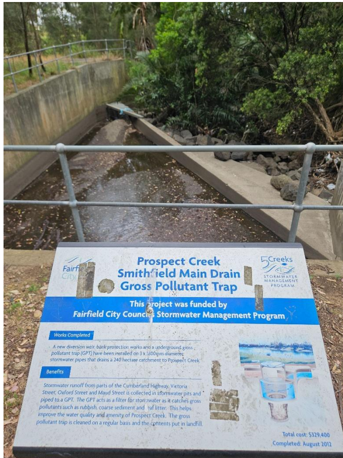
Photo Description: Gross Pollutant Trap Signage of Prospect Creek Smithfield Main Drain
