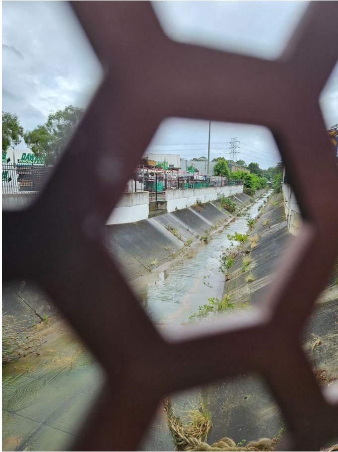
Photo Description: Stormwater culvert looking north from the road, some native tree growth.
