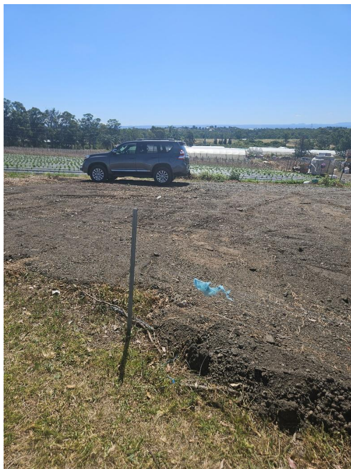
Photo Description: Intersection of Redmayne Rd and Ferrers Rd, facing south (high point)
