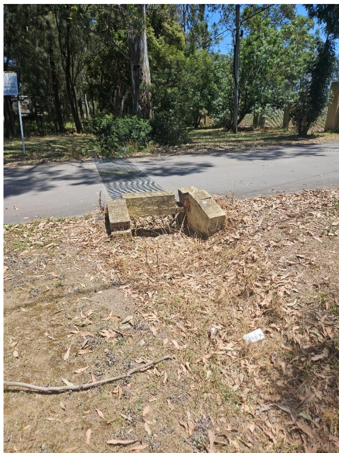
Photo Description: Drainage lines running east to Reedy Ck (east branch)
