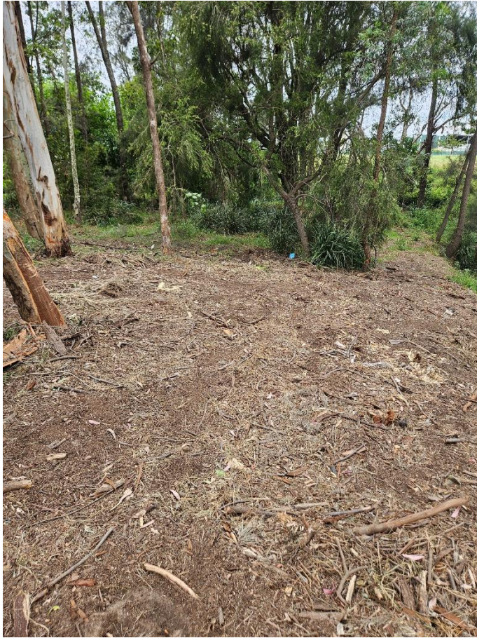
Photo Description: Vegetation clearing
