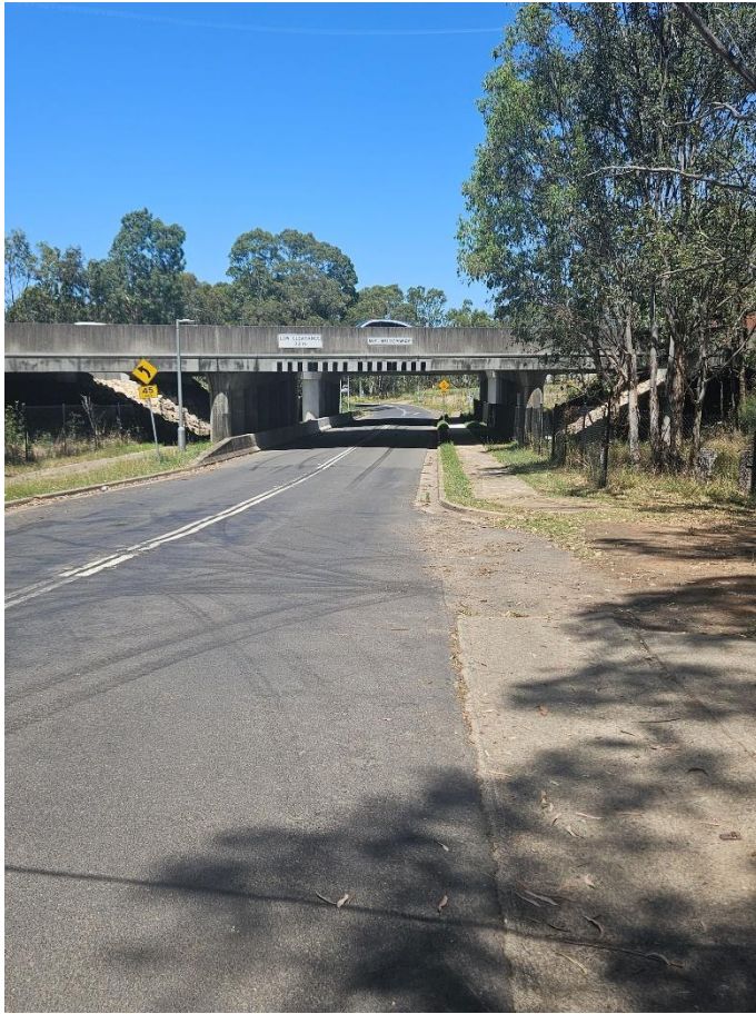
Photo Description: Underground services adjacent church
