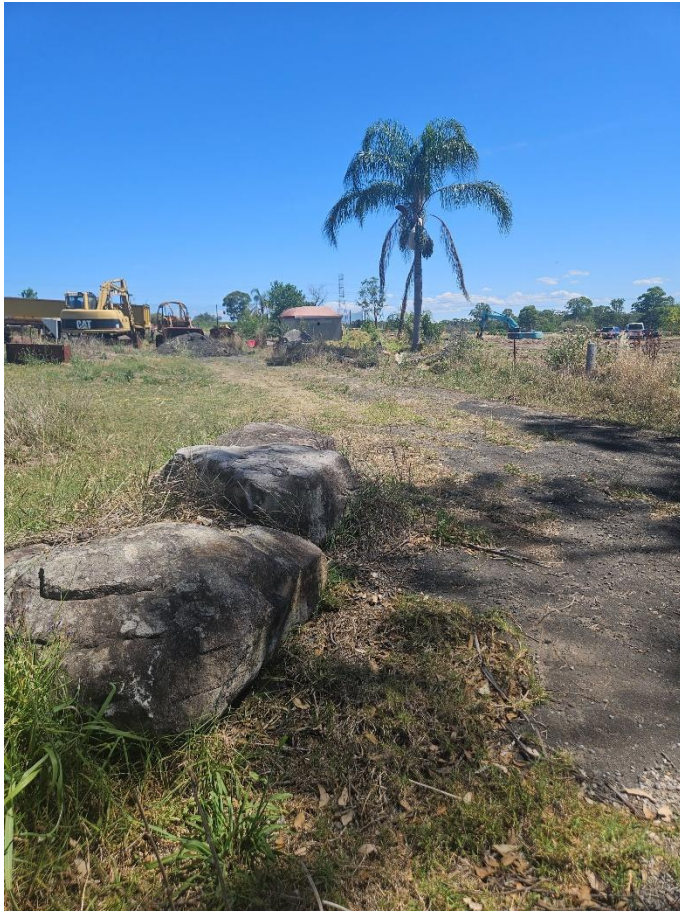
Photo Description: Construction works at an adjacent site
