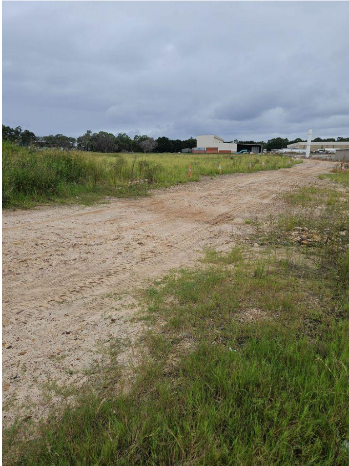
Photo Description: Vacant lot with cut and fill activities
