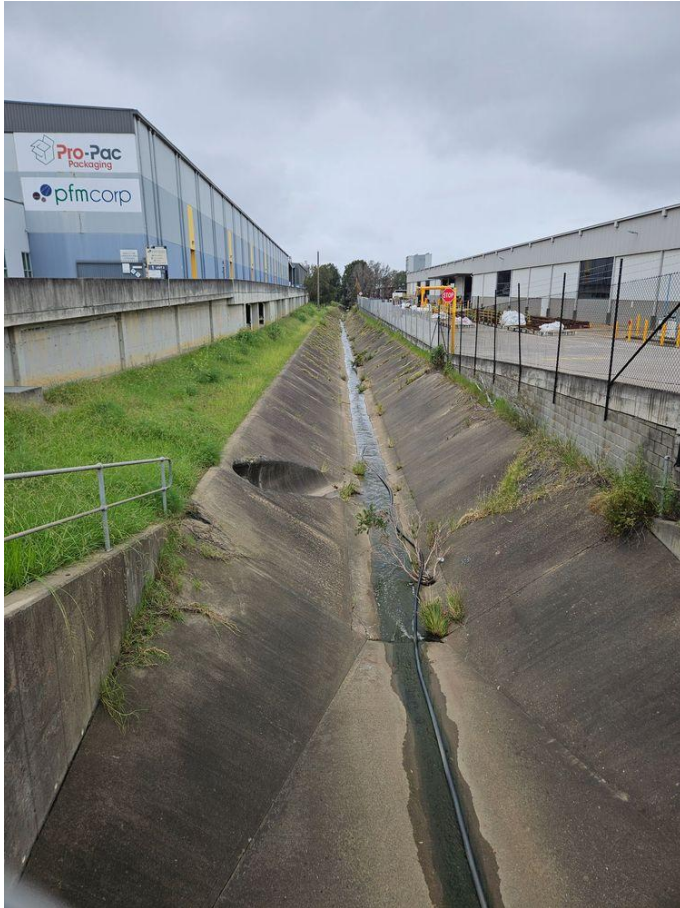
Photo Description: High velocity (but low flow) channel, flowing east, with stormwater culvert ingress.
