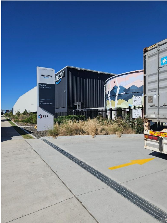
Photo Description: Transformer and retaining wall adjacent Amazon data centre and Johnston Cres, facing north at far southwestern corner of buffer
