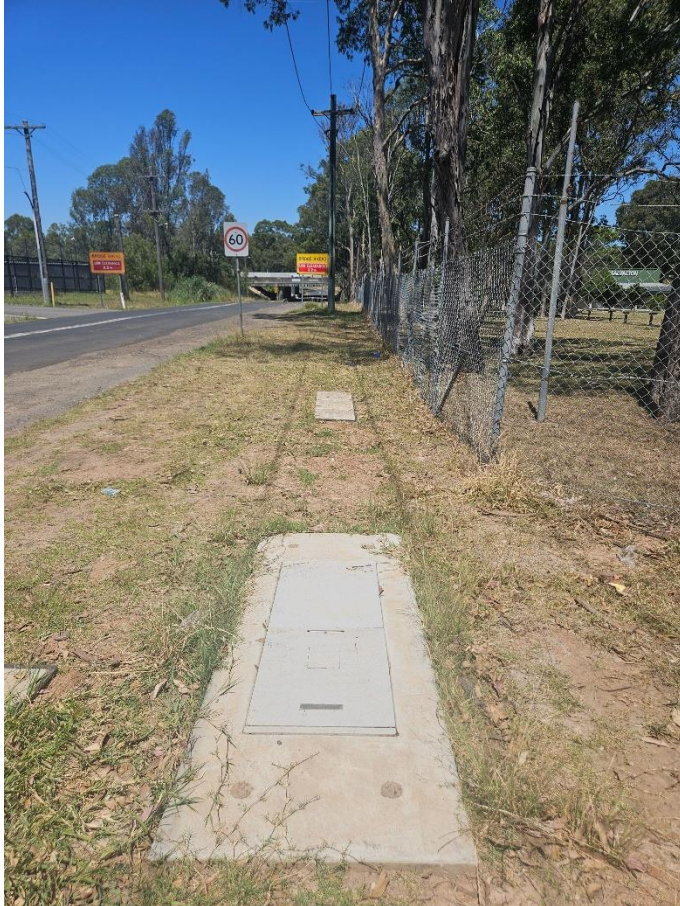
Photo Description: Drainage channel, Jemena gas pipeline, electricity Substations and Redmayne Rd with overpass for M7 motorway
