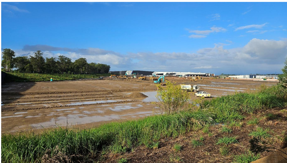
Plate 18. Substantial ground cutting and soil stripping at the western end of the Project Area. (Source: Heritage Now 2025)
