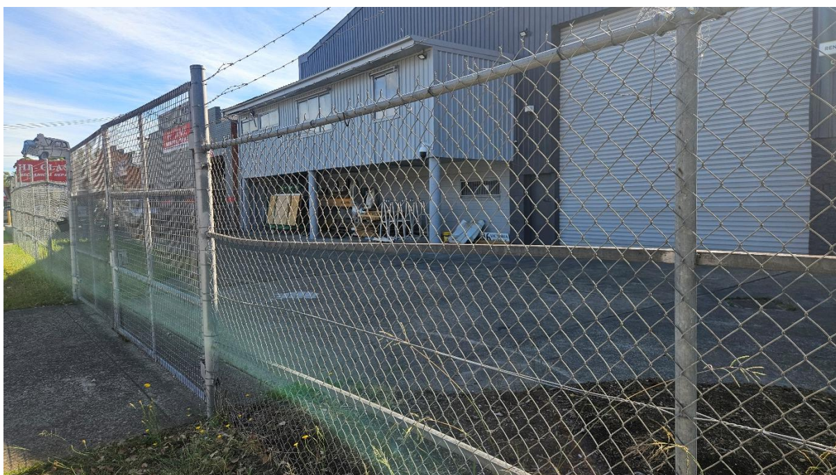
Plate 26. General view of the pump station location, facing north-east. (Source: Heritage Now 2025)
