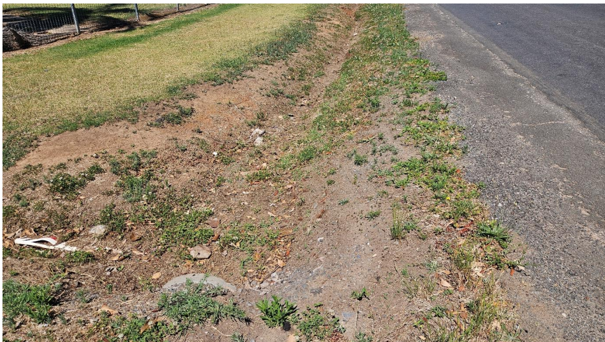
Plate 17. Example of a water culvert and a drainage channel next to the road. (Source: Heritage Now 2025)
