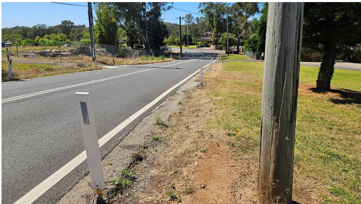
Plate 15. Example of road guide posts and electrical poles within the road verge. (Source: Heritage Now 2025)
