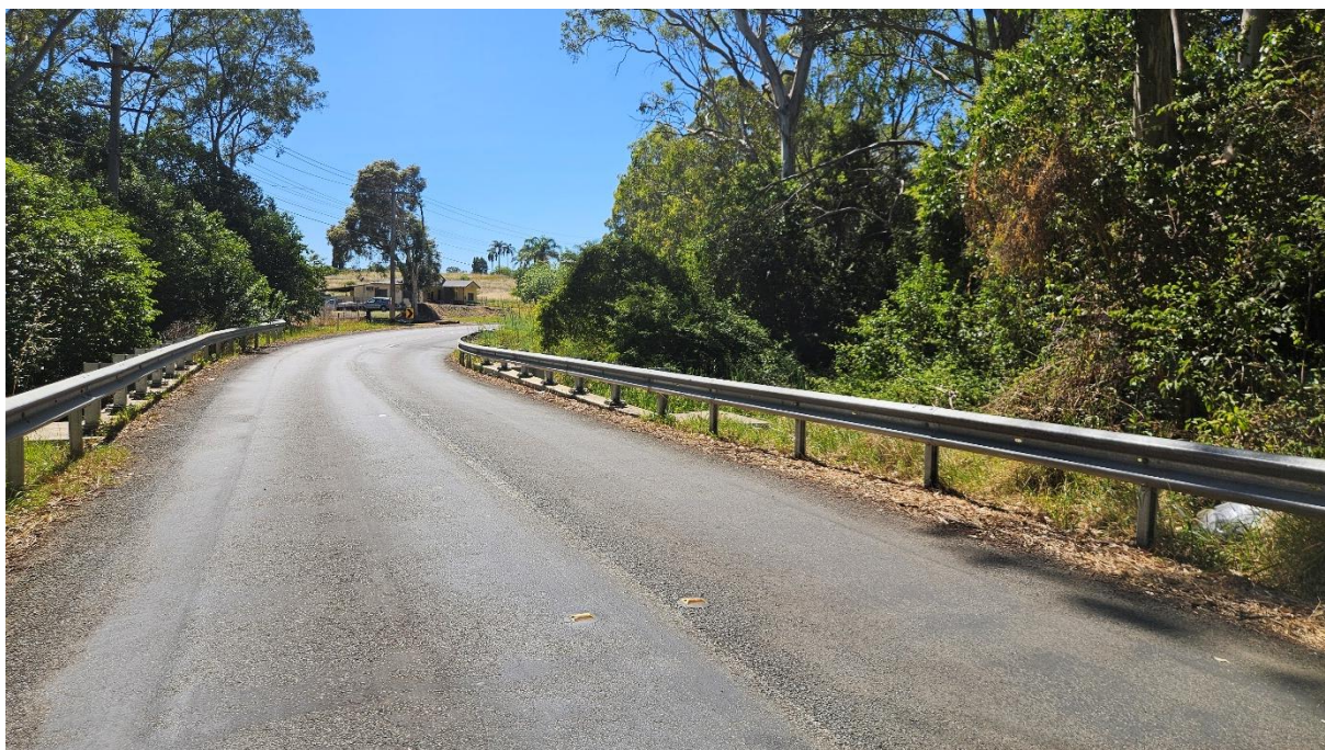
Plate 16. Metal safety railing installed next to the road. (Source: Heritage Now 2025)
