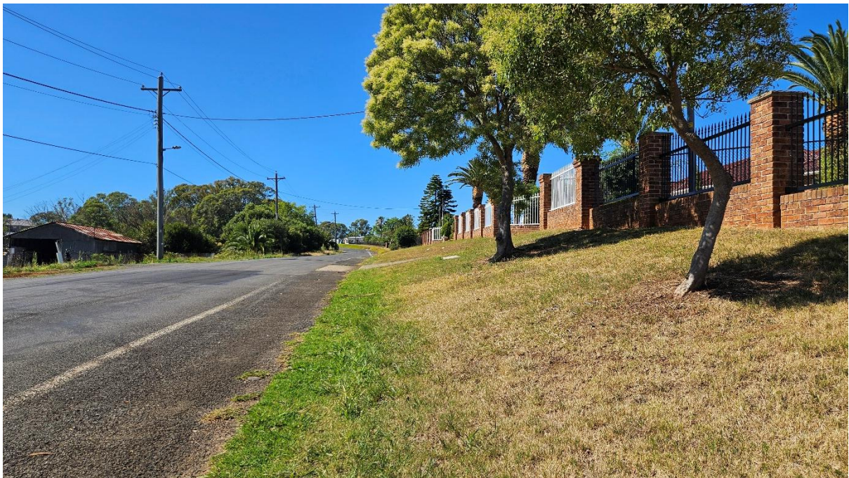
Plate 12. The natural landform has been cut through and modified for the construction of the road. (Source: Heritage Now 2025)
