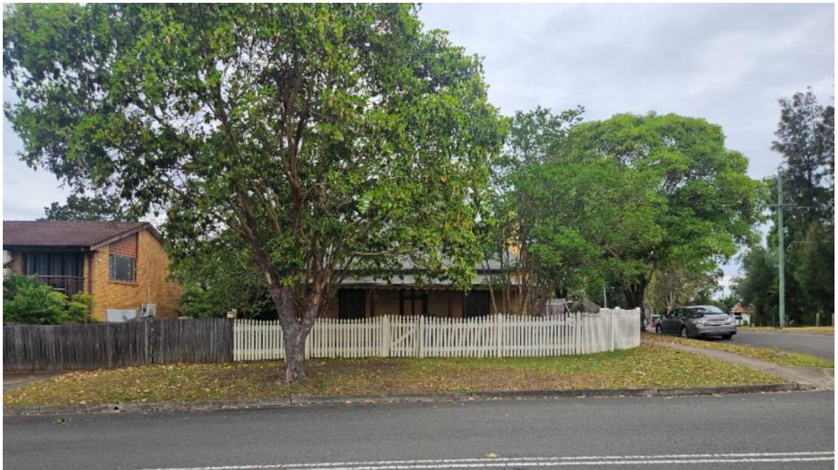
Plate 25. Direct line of sight between the Slab Cottage (188) and the Project Area, facing south. (Source: Heritage Now 2026)
