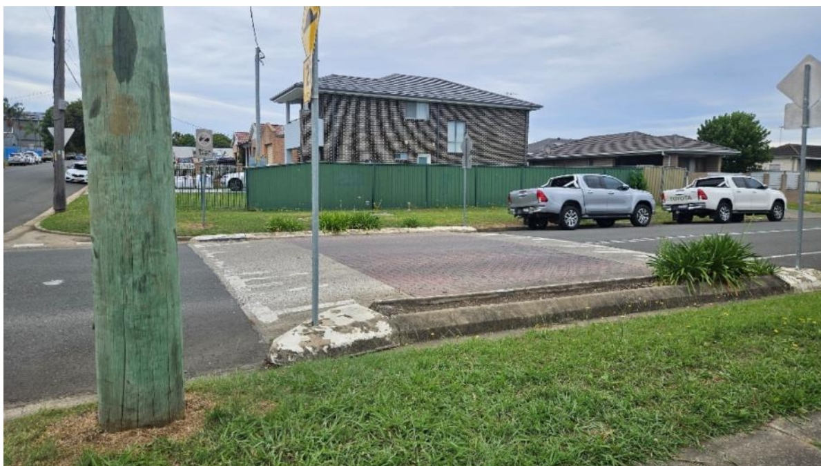
Plate 11. A speed reduction hump and a landscaped curb extension installed on an asphalt road within the Project Area. (Source: Heritage Now 2026)
