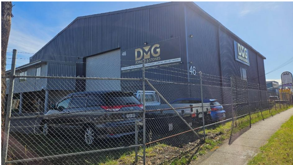
Plate 9. General view of the proposed pump station located at Victoria Street, facing north-east. (Source: Heritage Now 2026)
