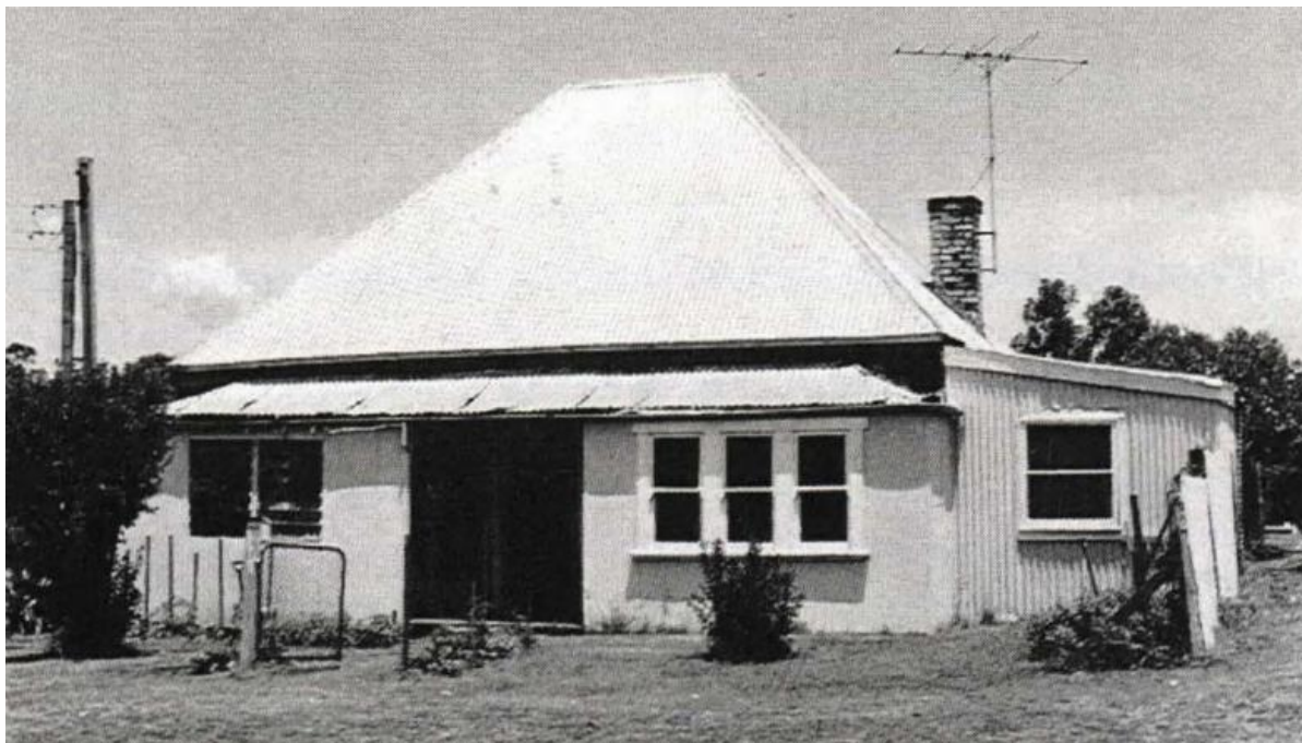
Figure 2. Photograph from 1992 heritage study showing enclosed front verandah and corrugated iron skillion, both since removed. (Source: Perumal Murphy Wu 1992, Ref. 051)
