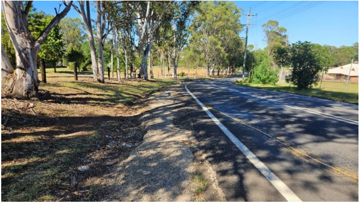
Plate 17. A portion of asphalted road meeting grass, within the western portion of the Project Area. (Source: Heritage Now 2026)
