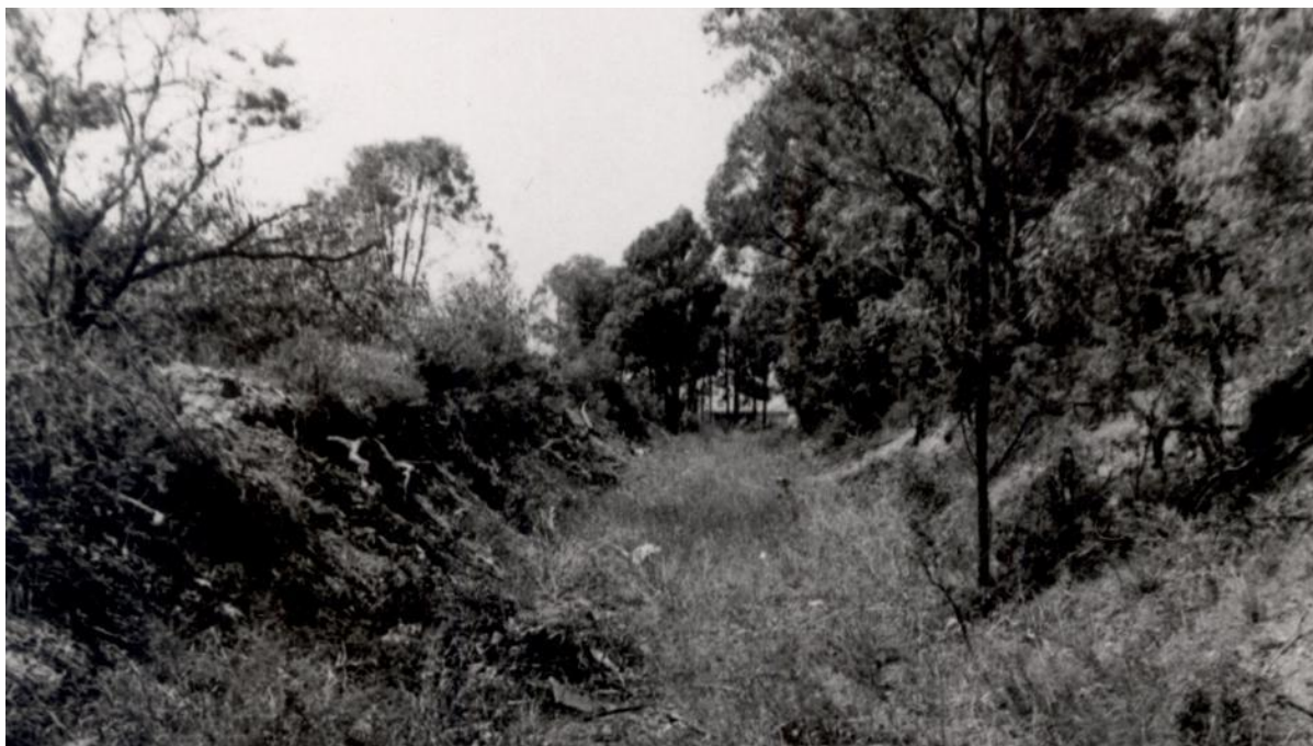
Figure 13. View north of the railway cutting for the Widemere Quarry line along the eastern side of Dublin Street, c.1978. (Source: Fairfield City Council Heritage Collection, HPC000133p)
