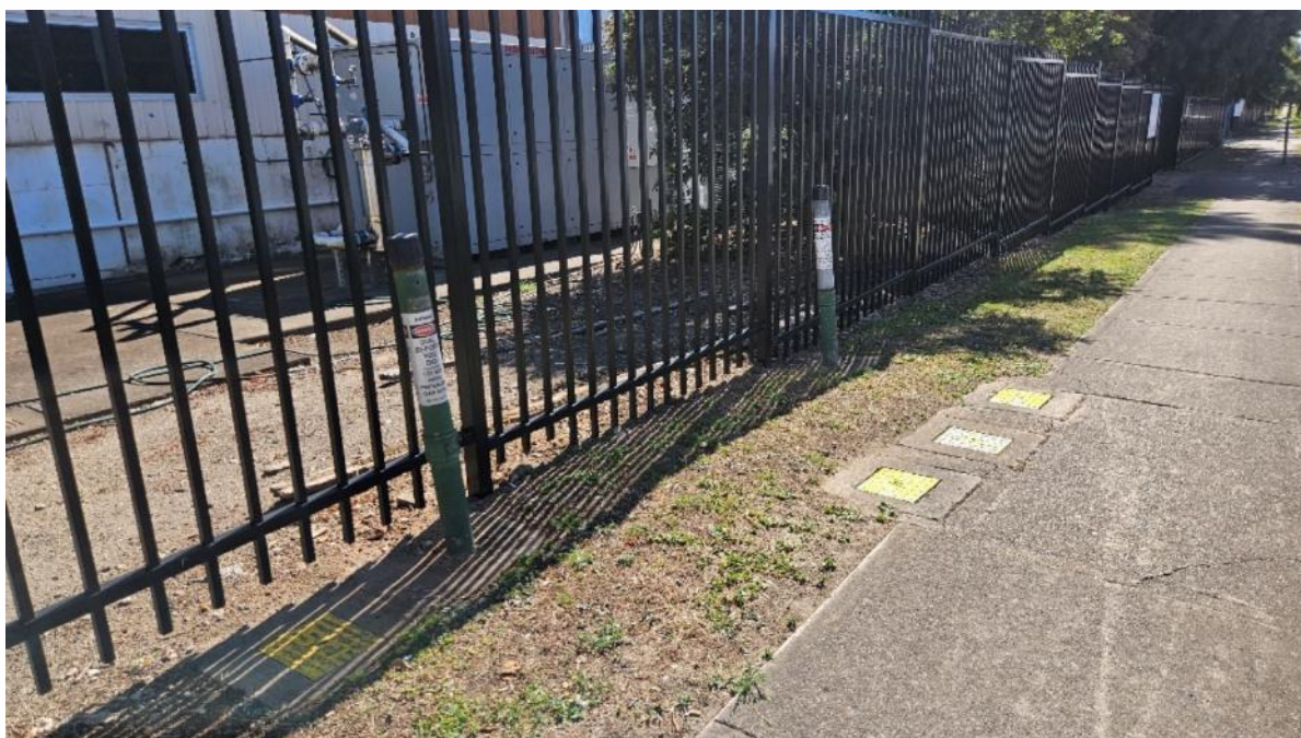
Plate 14. Example of services and a concrete pedestrian footpath within the road verge. (Source: Heritage Now 2026)
