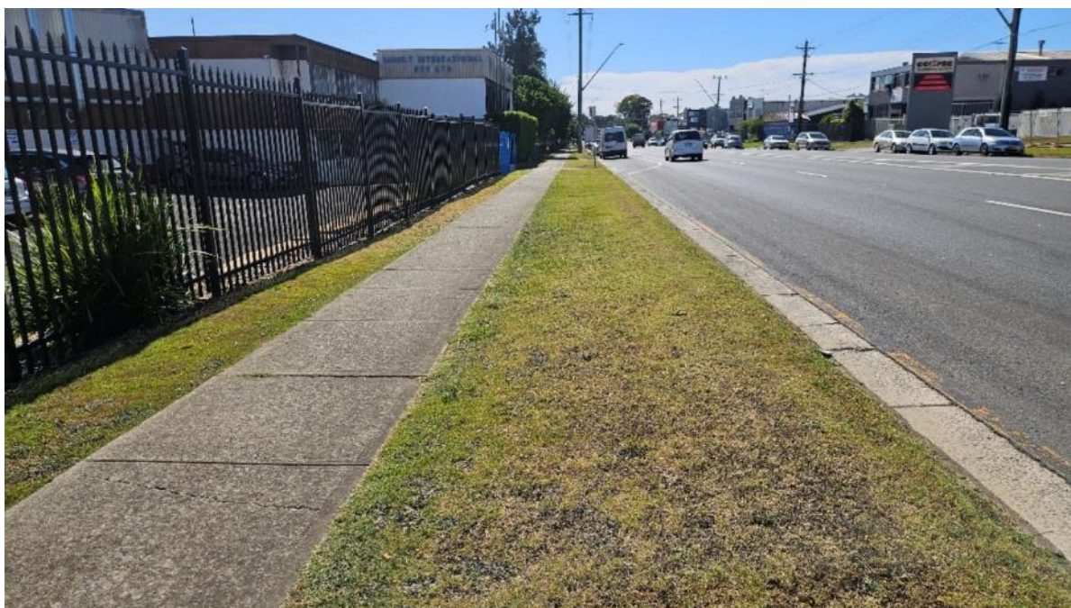
Plate 12. Example of a partially grassed and concreted road verge. (Source: Heritage Now 2026)
