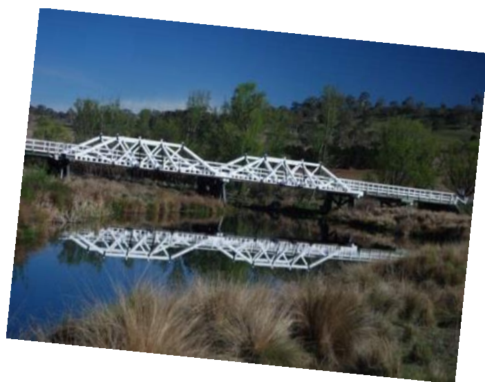
Coolumbooka River Bridge on the Bombala/Cathcart Road. One of the last remaining McDonald Truss Bridges in the State.
