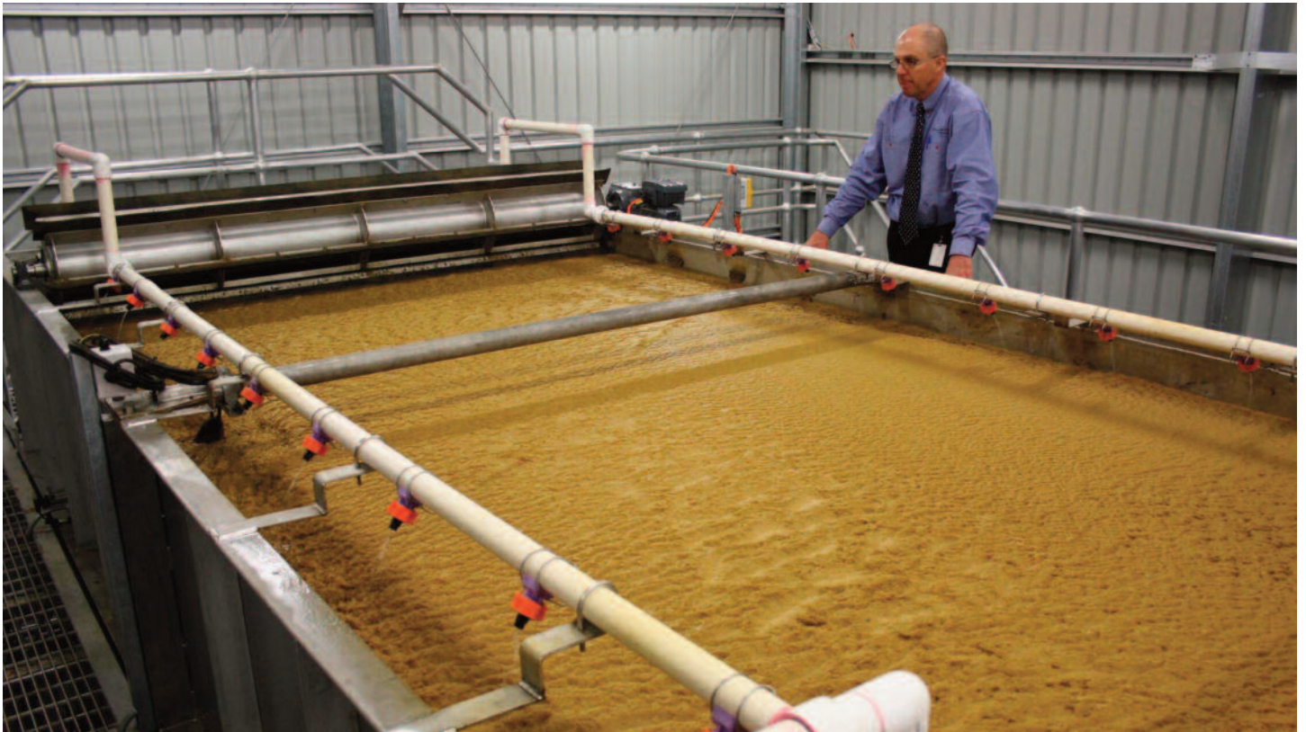
Flocculant Tank at the new Braidwood Water Treatment Plant (2014)
