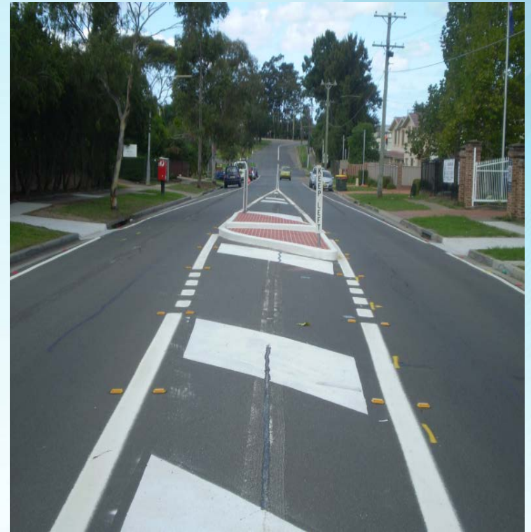
Banks Road, Heckenberg - new pedestrian refuge to improve pedestrian safety
