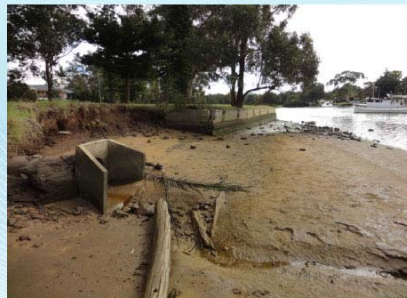
Stormwater outlet at Georges River at Pleasure Point to reduce overland flooding.
