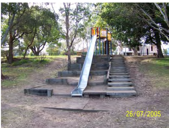
Playground equipment without any type of soft fall layer or other modern safety features. This equipment whilst still popular doesn't meet the latest safety standards and should be scheduled for removal and replacement.
