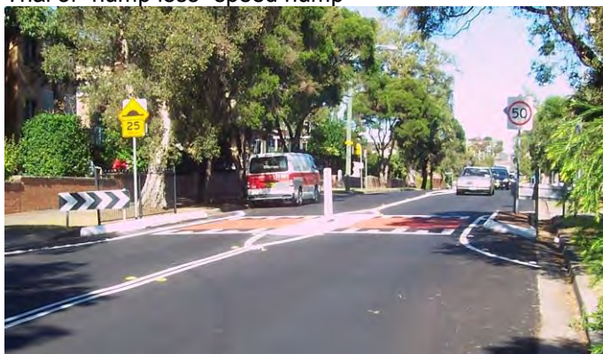
Trial of "hump less" speed hump
