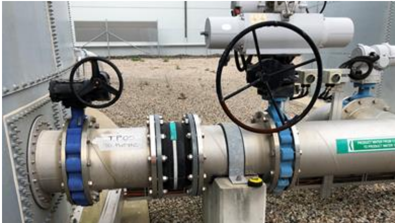
Figure 3. Existing PWT1 Inlet
