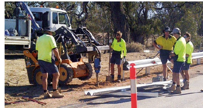
A damaged guard rail at Yarrein Bridge on the Swan Hill Road was replaced as part of routine maintenance and renewal work.
