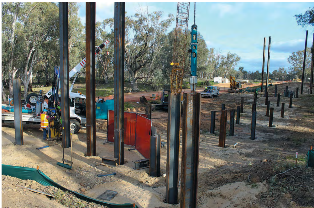
Column steel piles being installed for Nacurrie Road North Bridge.
