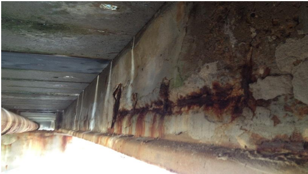
Candlagan Bridge Broulee – deteriorated and in need of replacement
