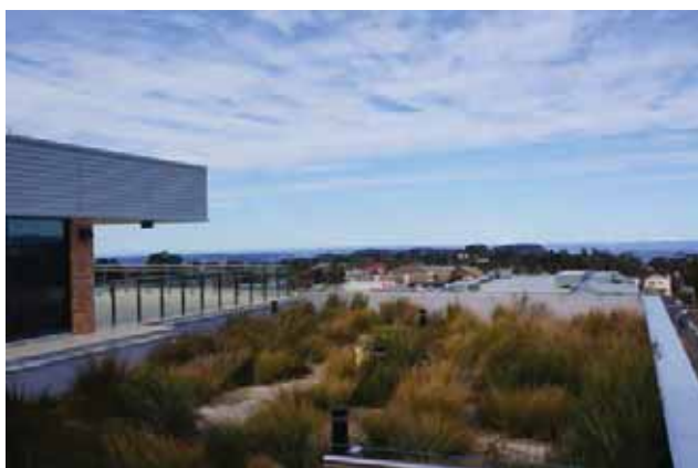
The green roof at the new Blue Mountains Cultural Centre (left) and the rain garden at Echo Point (right) treat and harvest stormwater for re-use onsite.
