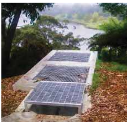
Gross pollutant traps, such as this one at Wentworth Falls Lake (left), capture and clean stormwater runoff from the surrounding streets, before it enters local creeks and waterways, including Wentworth Falls (right).
