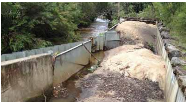
A Gross Pollutant Trap at Katoomba Falls prevents over 100 tonnes of sediment from entering the downstream World Heritage National Park every year.
