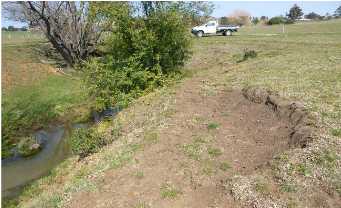
Photo 15: View looking at a back scarp in the creek bank in the northern part of the site..
