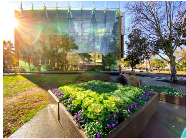
Image 3. Surry Hills Library, Crown Street
