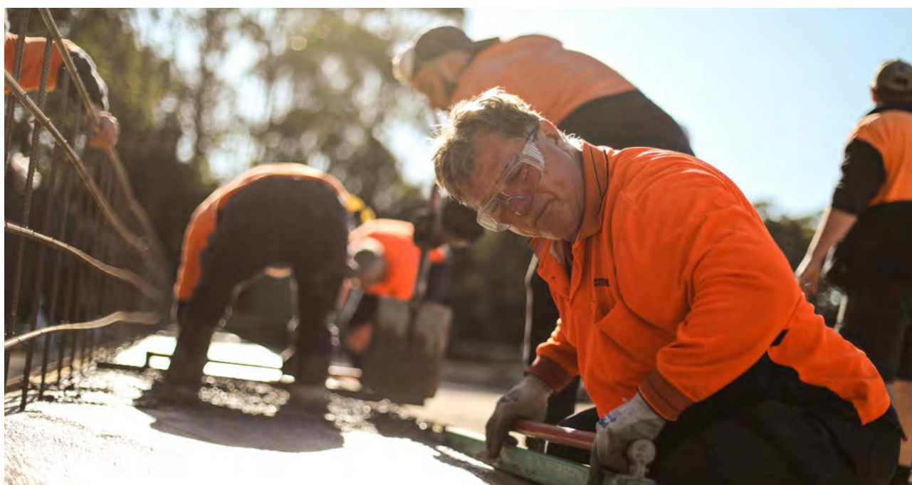
Image: Council staff renewing a footway
