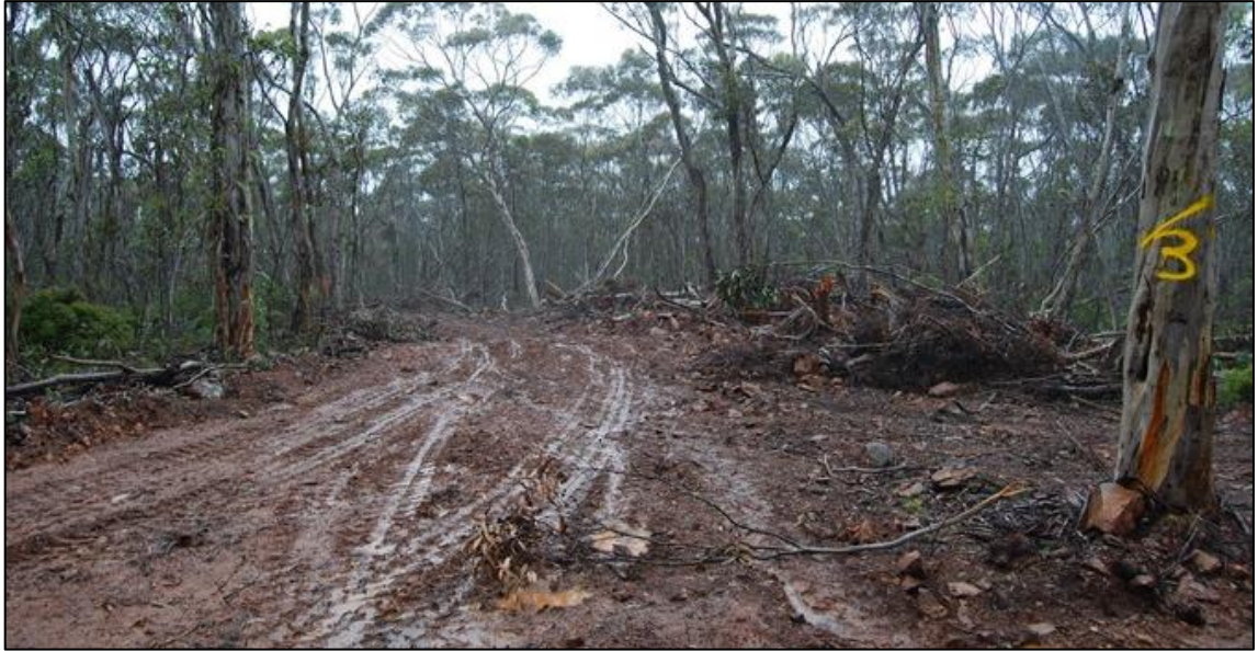
Plate A1: Road construction – track recently widened and drained
