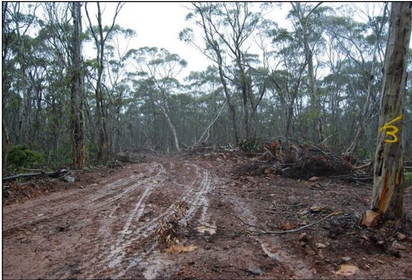
Plate 2-1: Road construction – track recently widened and drained
