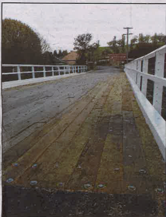
Naylor Street bridge, Carcoar, with its new wooden planks installed - it opened (unofficially) last week to traffic.
