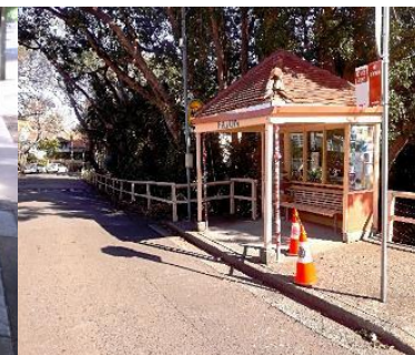
Poor/ Very poor:
