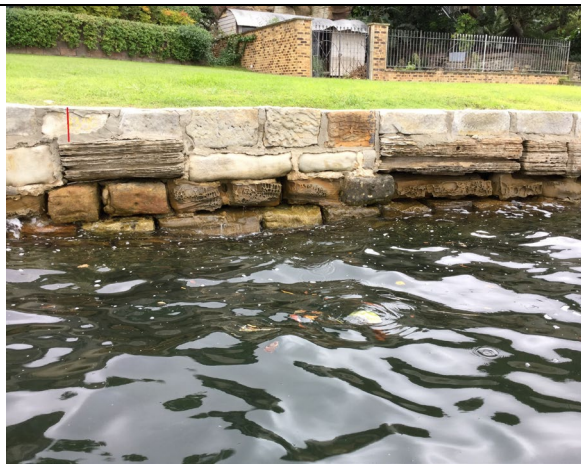
Seawall Grout Injection rehabilitation at Sawmillers Reserve — before
