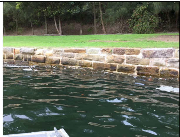
Seawall Grout Injection rehabilitation at Sawmillers Reserve — after
