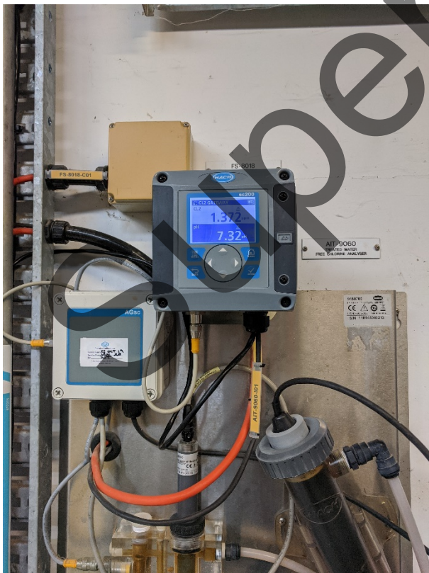
Figure 2-6 Treated water chlorine and pH analyser
