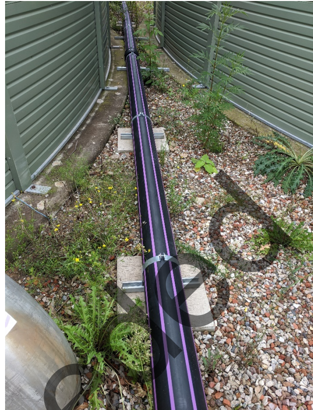
Figure 2-5 Off-spec divert pipe back to inlet works
