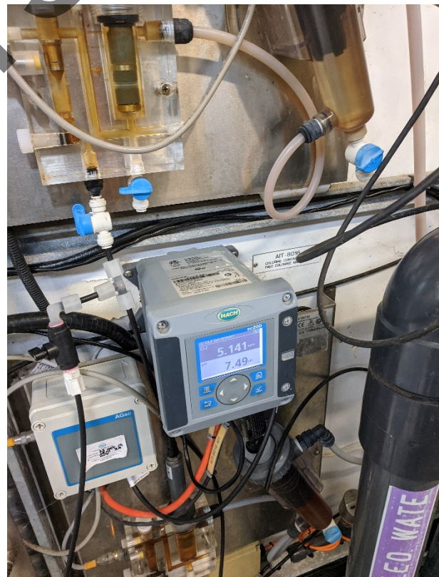
Figure 2-7 Chlorine contact tank chlorine and pH analyser
