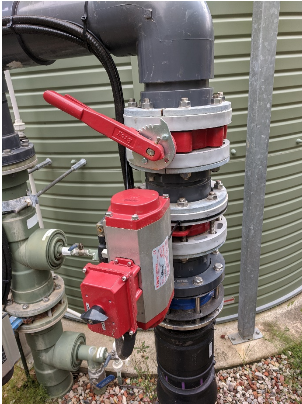
Figure 2-4 Off-spec divert pipe valve
