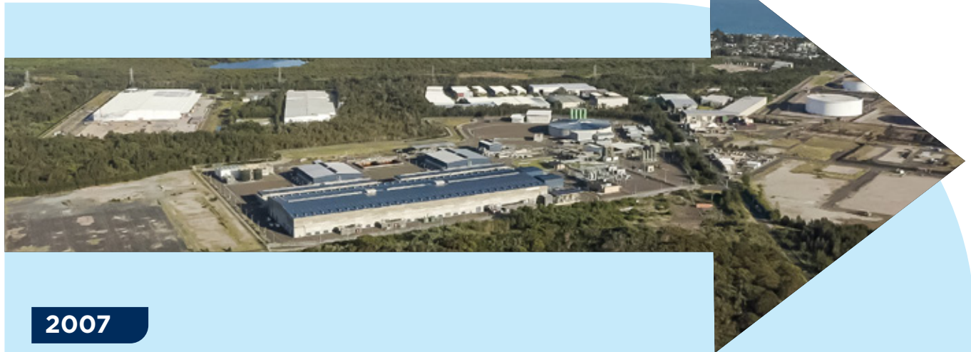
Figure 10: The history of the Sydney Desalination Plant
