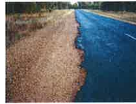
Existing Edge Breaks on Sealed Road
