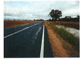
Edge Breaks after Widening and Reseal
