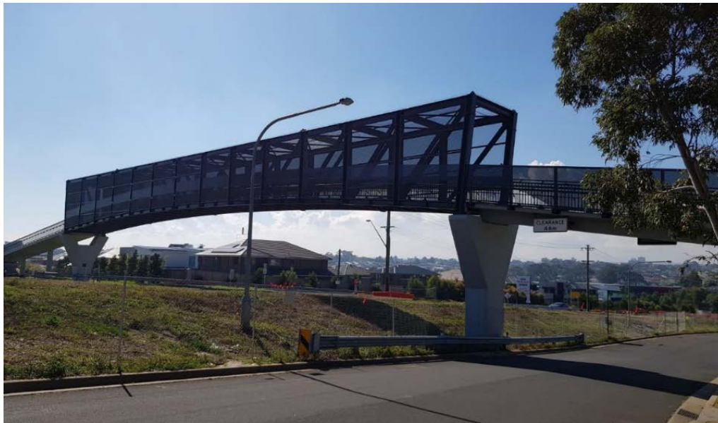
Figure 2.1 Existing pedestrian bridge at Pellizzer Boulevard
