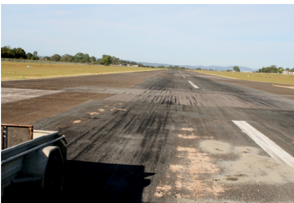
Patching potholes in the Taree airport runway
