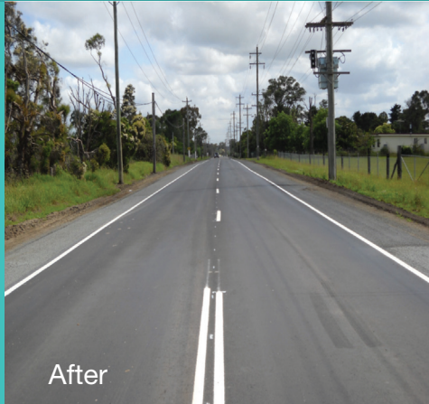
Heavy patching, reconstruction and resurfacing to restore failed pavement at Devonshire Road, Kemps Creek
