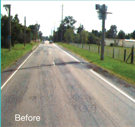
Heavy patching, reconstruction and resurfacing to restore failed pavement at Devonshire Road, Kemps Creek
