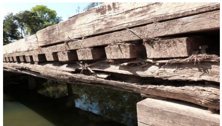
Browns Bridge on Browns Crossing Road
