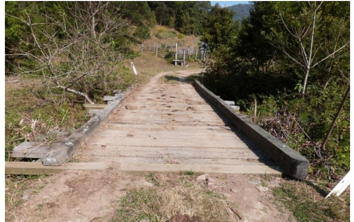
Menzies Bridge on South Arm Road
