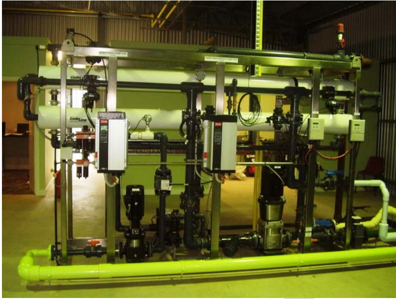
Figure 4, Existing UF membrane unit at Deep Creek Resort (Moama NSW)
