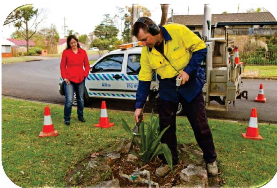
Figure 7 Acoustic equipment is used to actively detect leaks, so they can be repaired.
