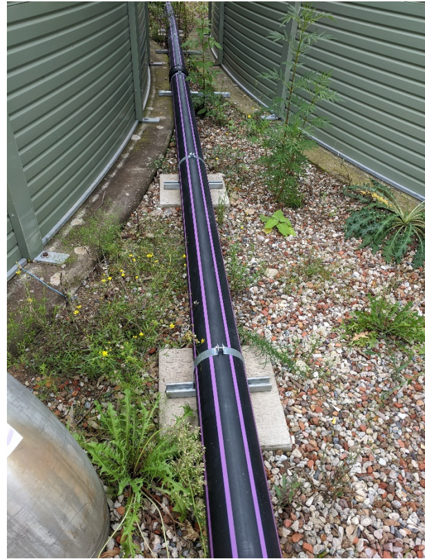
Figure 2-5 Off-spec divert pipe back to inlet works
