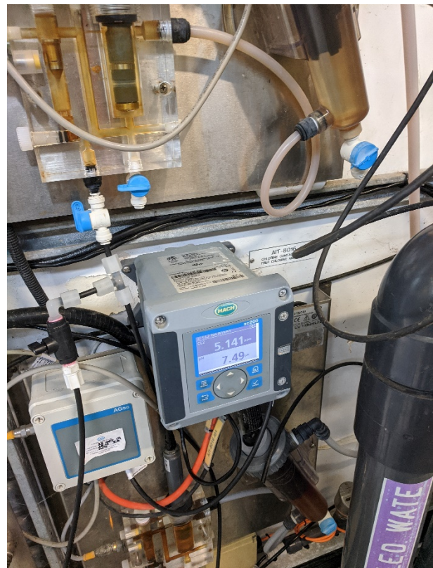
Figure 2-7 Chlorine contact tank chlorine and pH analyser
