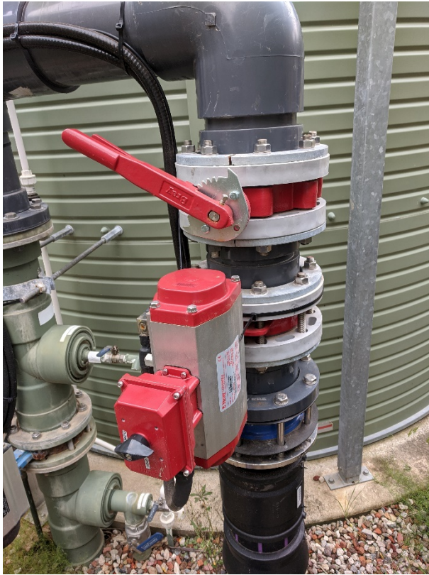
Figure 2-4 Off-spec divert pipe valve
