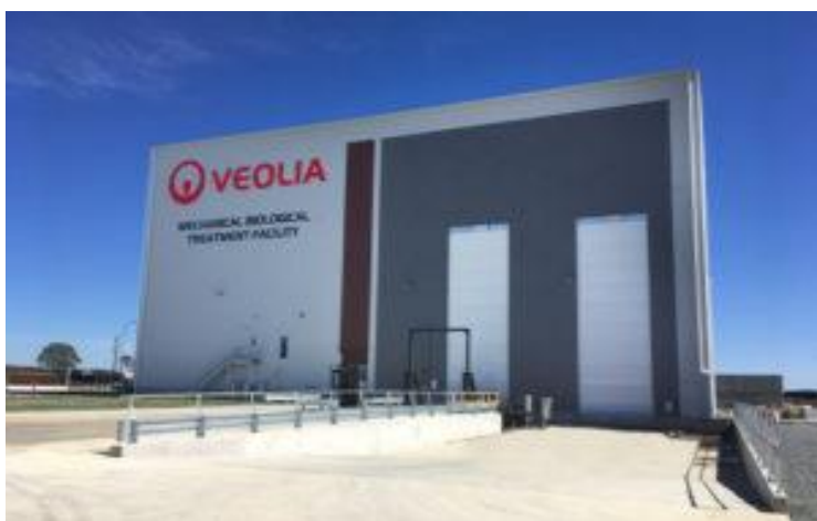
Figure 2: Veolia MBT facility located at Woodlawn.
