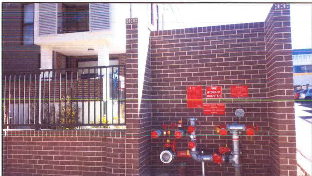
Figure 7 - Tank suction booster assembly serving a Class 2 building
