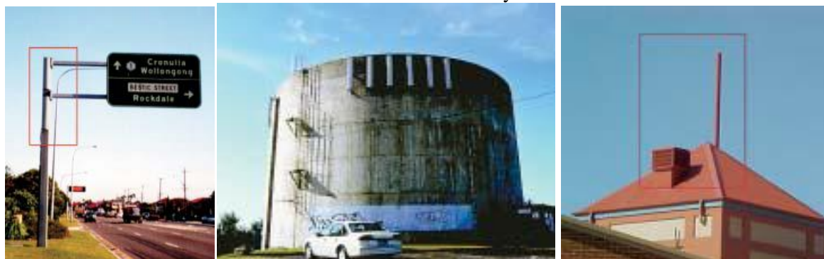
-Panel antennas co-located on a road sign -Co-location on a water tank
