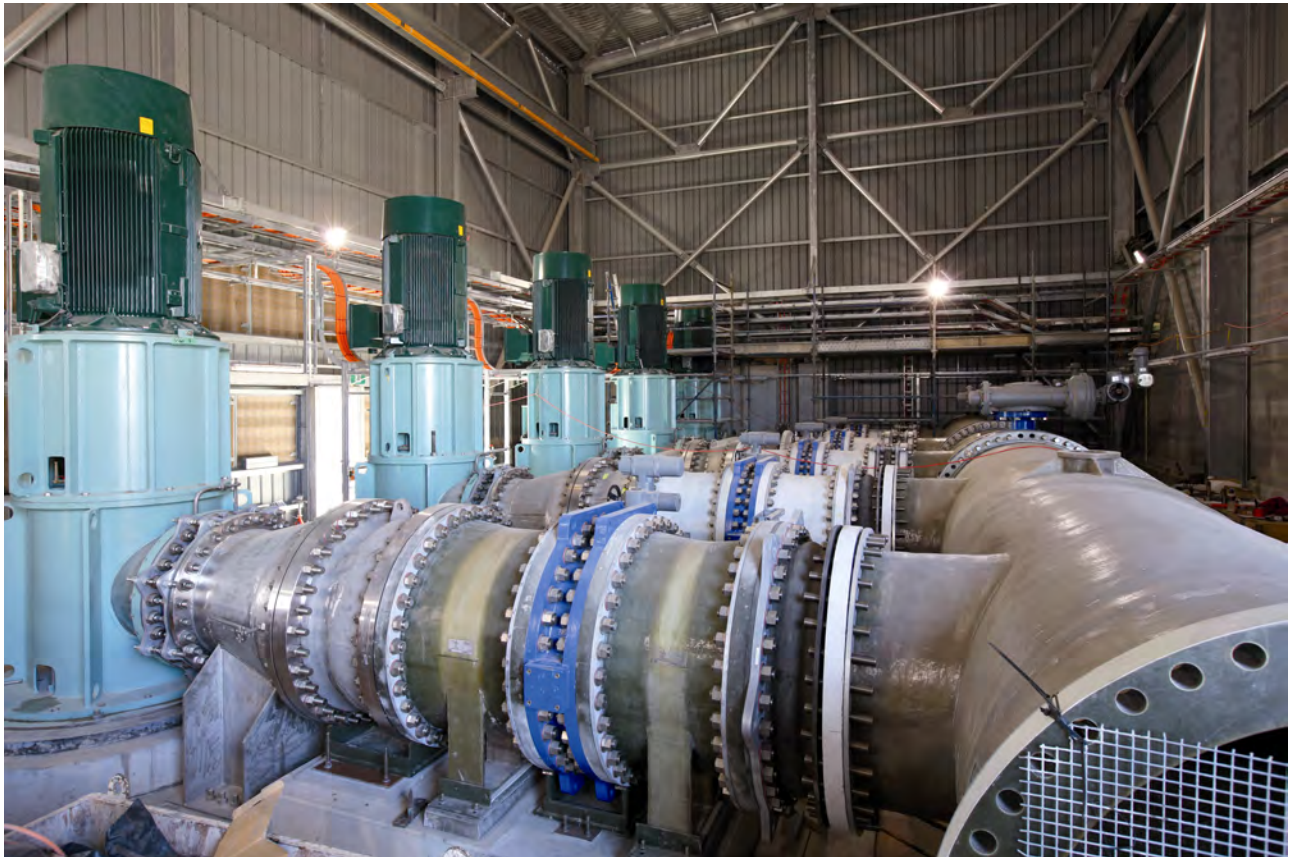
Figure 1.3 Pumps in the desalination plant's drinking water pumping station
