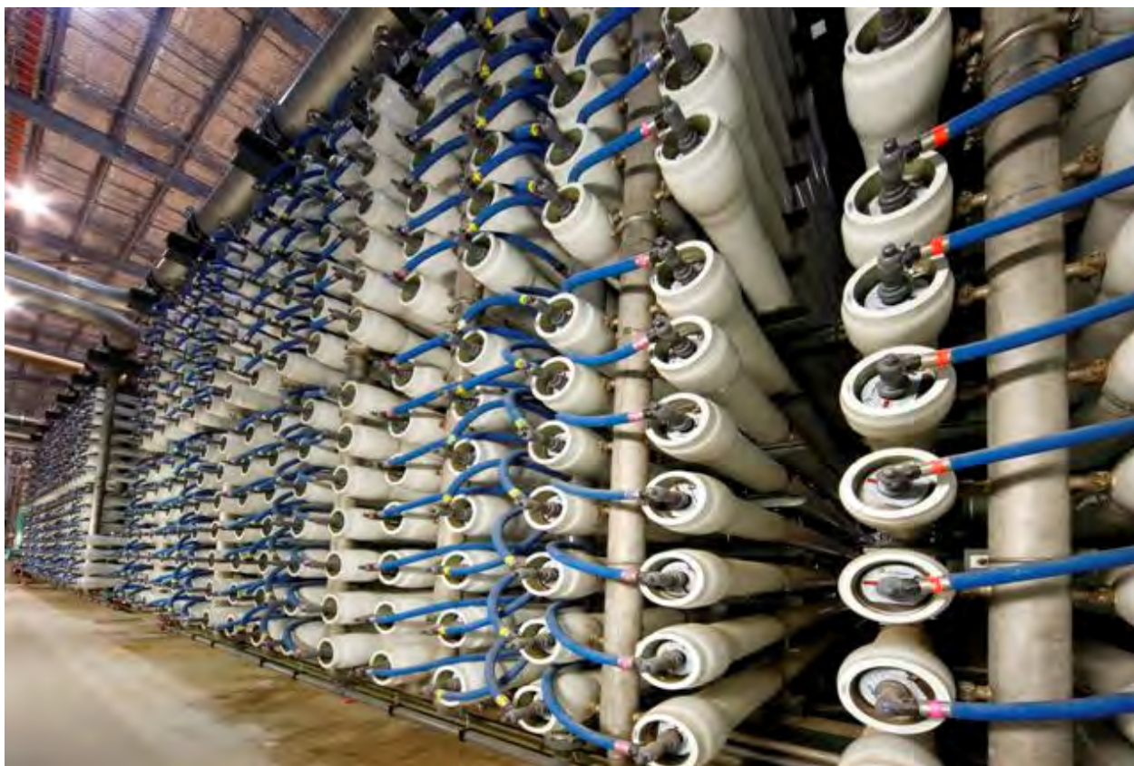
Figure 3.1 Reverse osmosis membranes in the desalination plant.
