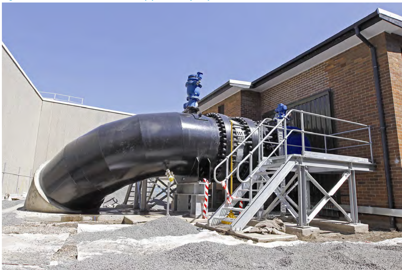
Figure 4.1 Connection of the bulk water pipeline to Sydney Water's network.
