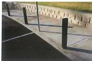
Subsurface fixed rectangular timber bollard
