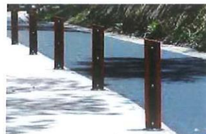
Surface fixed rectangular timber bollard
