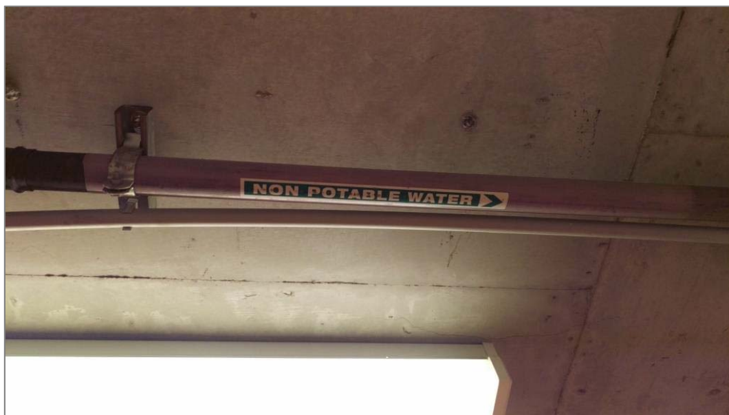
Figure A.6.2 Recycled water pipework coloured lilac and appropriately labelled.
