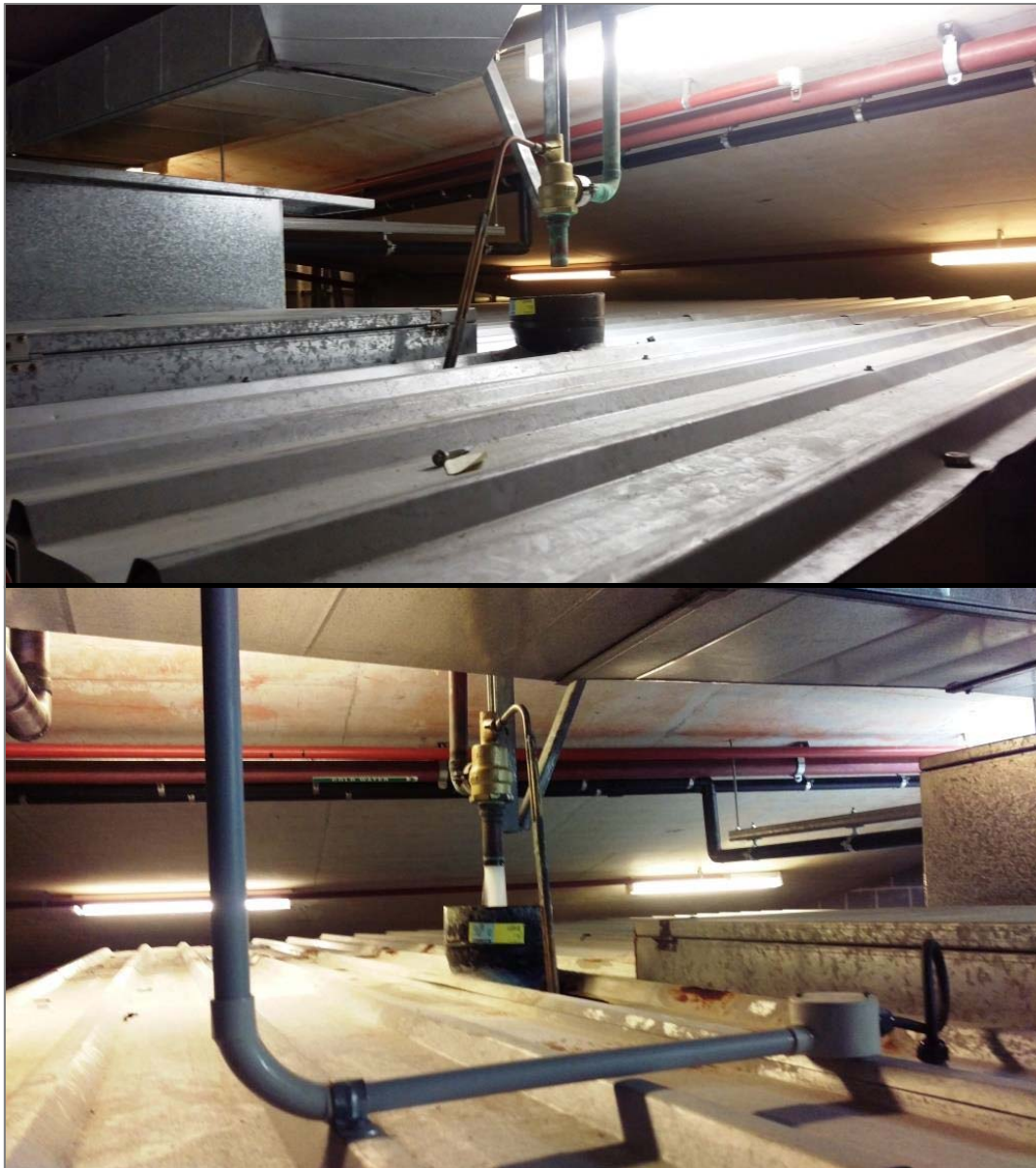
Figure A.3.6 Potable water supply used for top-up of the recycled water storage tanks is protected by air gaps (as well as an RPZD backflow prevention device). Note top-up in operation in bottom view.
