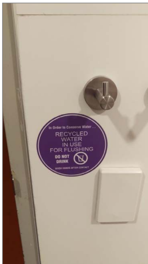
Figure A.6.3 Recycled water labelling in toilet facility (located on wall adjacent to door). It was noted that there were no hose bibs in the toilet areas inspected.
