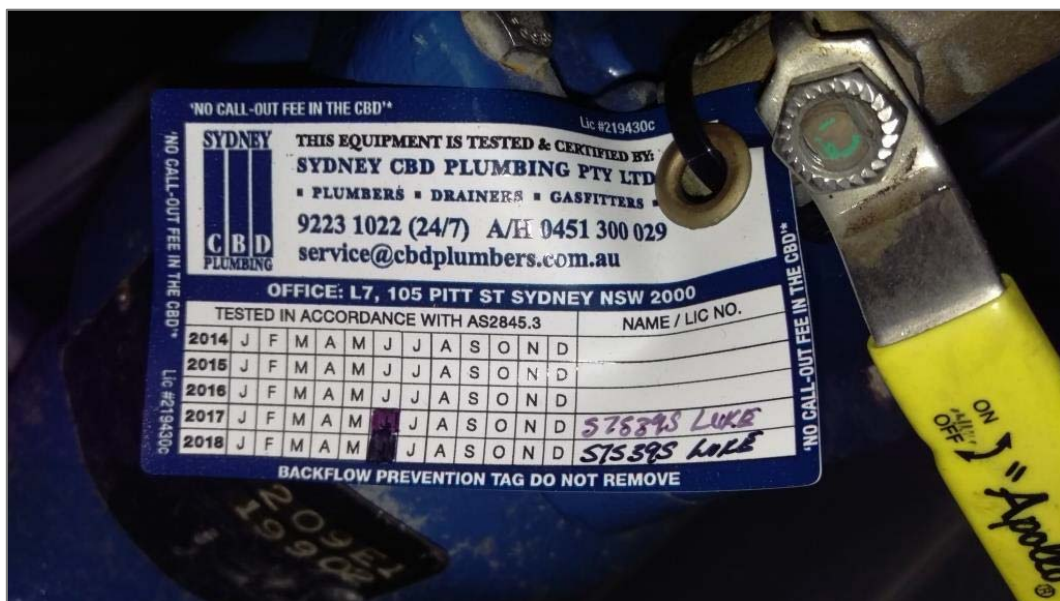
Figure A.3.5 RPZD backflow prevention devices are tested annually.
