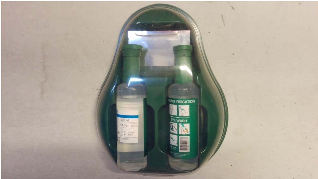
Figure A.3.2 Readily accessible eye wash facilities located adjacent to chemical storage areas.
