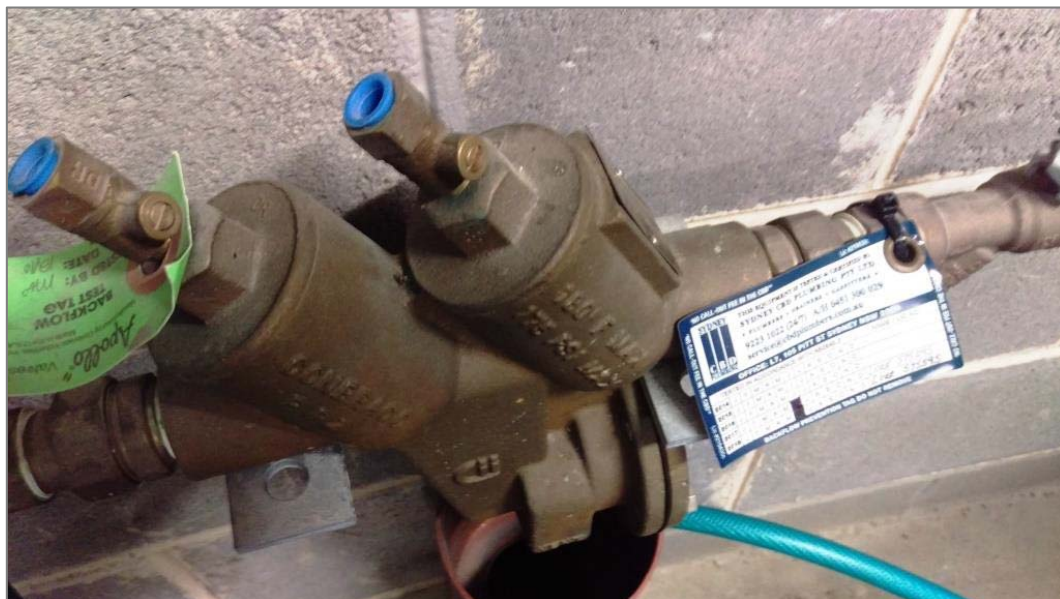
Figure A.3.4 Potable water supply used for top-up of the recycled water storage tanks is protected by an RPZD backflow prevention device (as well as air gaps).
