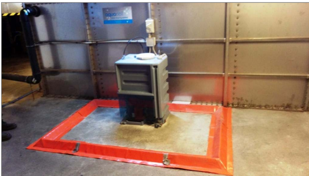
Figure A.3.1 Bunding around chlorine solution storage container, which is located adjacent to the chlorine contact/finished water tank.
