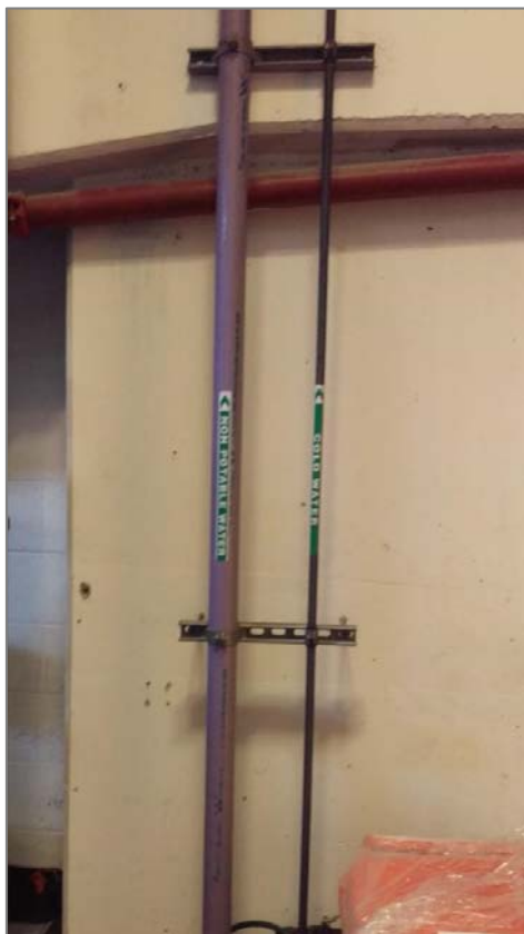
Figure A.6.1 Recycled water pipework coloured lilac and appropriately labelled.
