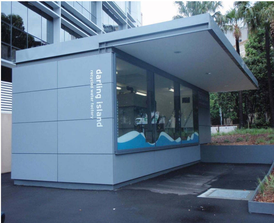
Photograph 1 Darling Harbour Water Recycling Facility
