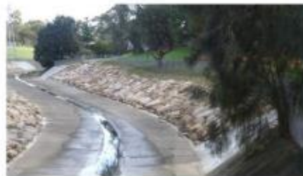
Immediately after - less steep sandstone lined banks with new seedlings
