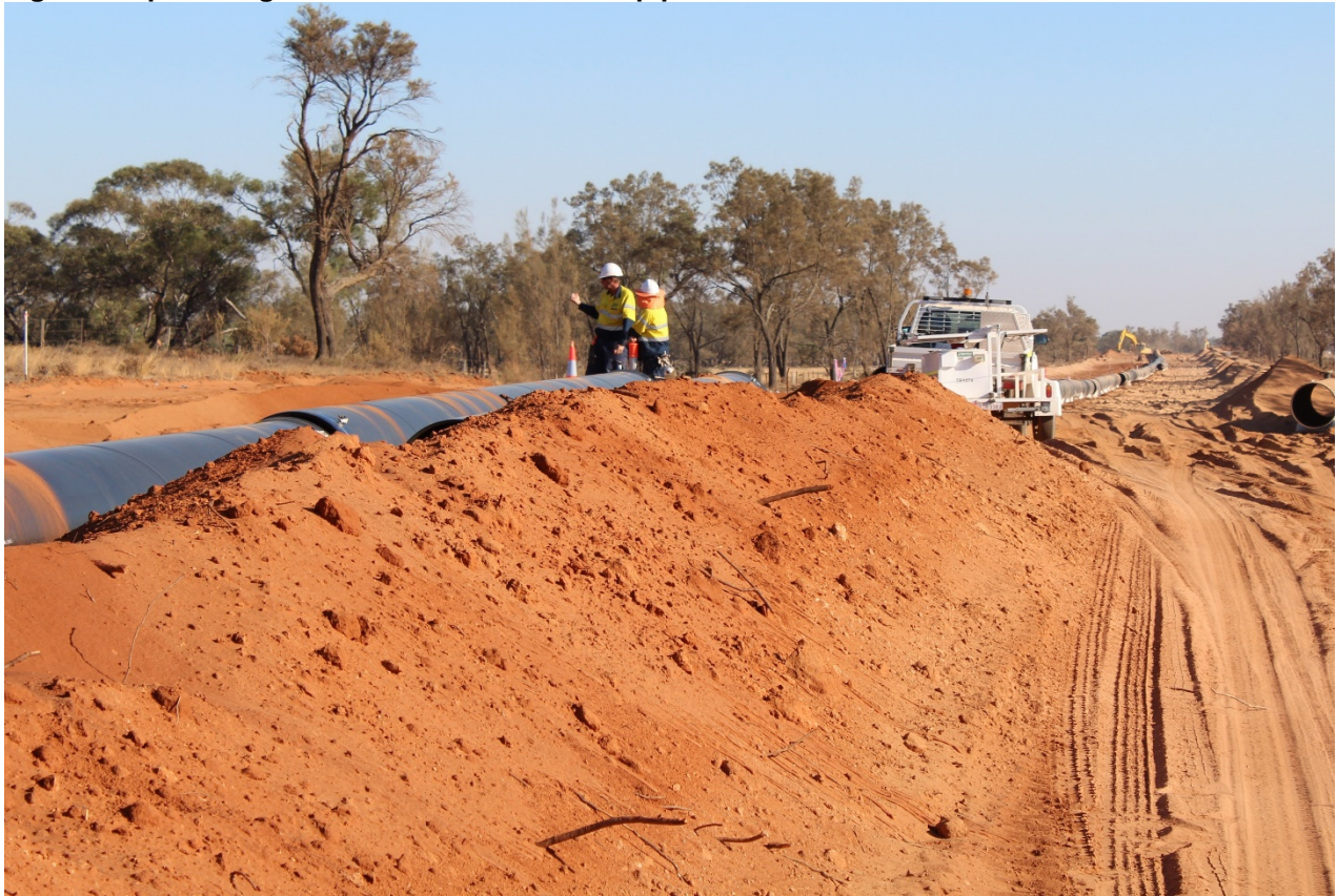
Figure 8 Pipe strung at the southern end of the pipeline route
