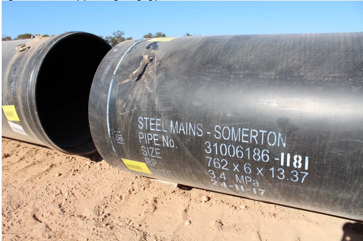
Figure 10 Picture of pipe during stringing process
