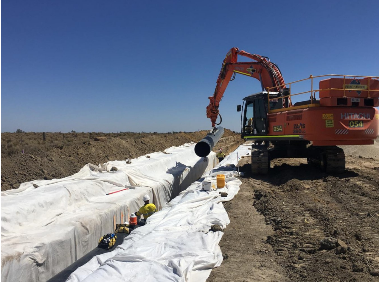
Figure 11 Machine laying pipe
